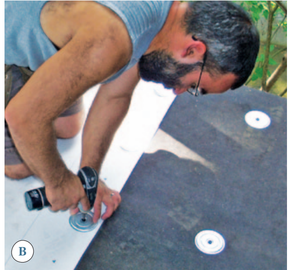
Figure 3. Cutouts in the membrane (A) allowed it to slip over the tops of the posts, minimizing seams; an open cutout at the outside corner column accommodates the membrane turn-down along both edges. The upper edge of the first sheet of membrane is screwed to the deck at 12-inch intervals. A preprinted line 4 inches from the edge marks the correct overlap for the next sheet (B). Turned-down membrane edges are secured to the PVC fascia with double-sided tape approved by the TPO manufacturer (C).
