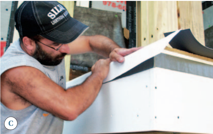
Figure 3. Cutouts in the membrane (A) allowed it to slip over the tops of the posts, minimizing seams; an open cutout at the outside corner column accommodates the membrane turn-down along both edges. The upper edge of the first sheet of membrane is screwed to the deck at 12-inch intervals. A preprinted line 4 inches from the edge marks the correct overlap for the next sheet (B). Turned-down membrane edges are secured to the PVC fascia with double-sided tape approved by the TPO manufacturer (C).
