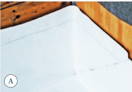
Figure 4. Because seams at inside corners leave a potential pinhole leak where the deck and walls intersect, a prefabricated corner piece is heat-welded to all three surfaces (A, B). Peel-and-stick membrane flashing adhered to the sheathing (C) will later be covered with housewrap.
