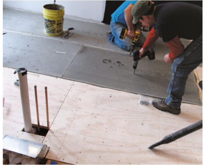
Figure 4. Carpenters troweled thinset onto a layer of 1/2-inch plywood installed over the AdvanTech sheathing (above left), then screwed down 1/4-inch backerboard (above). The surface was skim-coated and edged with dams and a perimeter expansion joint in preparation for electric heat mats and self-leveling underlayment (left).
