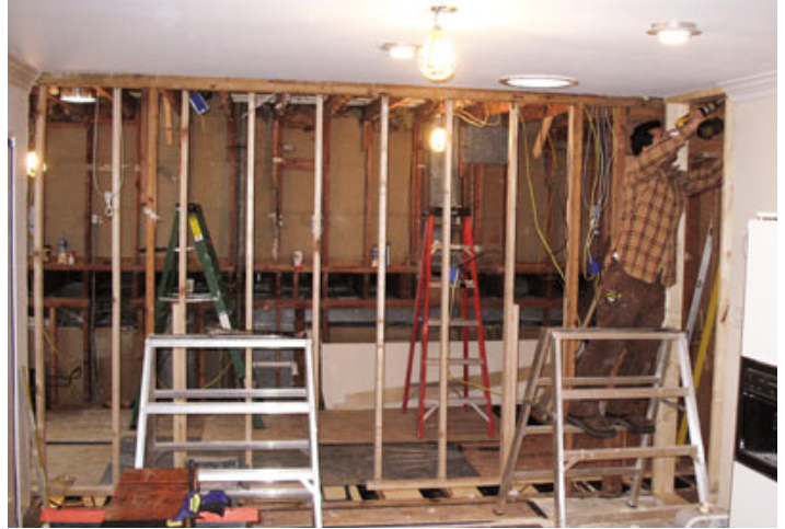
Figure 1. In the original floor plan, a bearing wall separated the dining room from the kitchen (left). The first step in combining the two spaces was to provide temporary support for the ceiling and remove the wall in preparation for installation of a flush beam (right).
