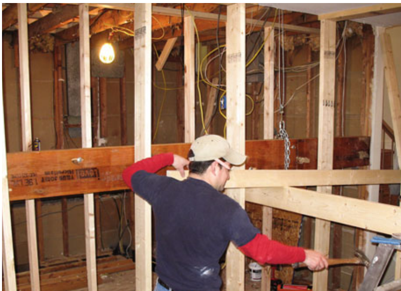
Figure 2. The double-LVL and steel fitch beam was fastened together with 1/2-inch-diameter bolts 16 inches on-center (top). A pair of come-alongs rigged in the attic helped hoist it into place (above). Each end of the beam was supported by a 4-inch-by-6-inch Parallam column (right).
