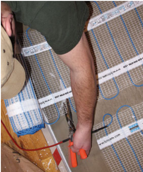
Figure 5. Laticrete's electric heat mats are designed to be cut to fit in the field (left) and have a self-adhesive backing that holds them in place; tape and thinset are also useful to hold down edges and wiring connections. While the mats can be covered with thinset, the author prefers to use a self-leveling underlayment (right).
