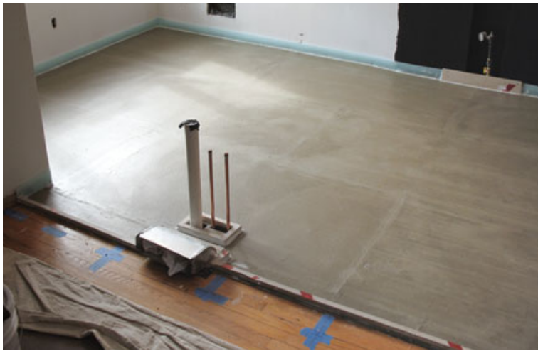
Figure 4. Carpenters troweled thinset onto a layer of 1/2-inch plywood installed over the AdvanTech sheathing (above left), then screwed down 1/4-inch backerboard (above). The surface was skim-coated and edged with dams and a perimeter expansion joint in preparation for electric heat mats and self-leveling underlayment (left).
