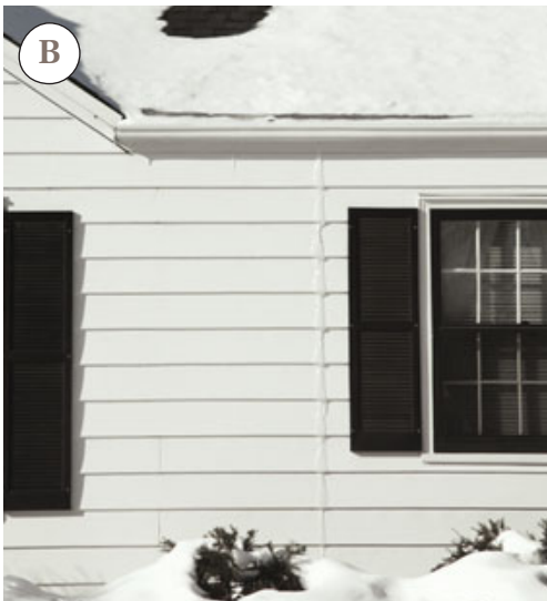
Figure 2. Ice dams form on cold days when heat leaking from inside the home warms the attic enough to melt the snow on the roof (A). Damaging leaks may show up in subtle ways, like this line of ice emanating from behind the siding (B), or not so subtly, in the case of icicles growing out of a soffit (C). Tannin stains on the siding of this home (D) are unmistakable evidence that lumber in the structure is being drenched with snowmelt.
