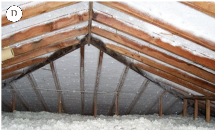
Figure 4. Uninsulated can lights are a common source of attic heat (A). Leaks around bath ceiling fans (B) introduce moisture as well as heat, as evidenced by mold on the sheathing in this attic. In one home, a disconnected vent pipe led to icicles inside the attic as well as ice dams on the roof (C). Frost can build up in the attic even when there is no ice on the roof (D); this is an insidious problem, as it can take weeks to detect.
