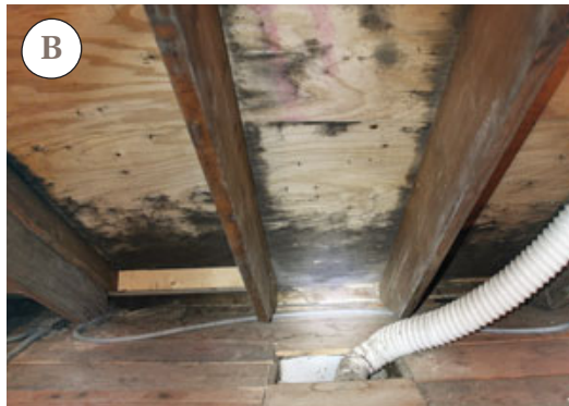
Figure 4. Uninsulated can lights are a common source of attic heat (A). Leaks around bath ceiling fans (B) introduce moisture as well as heat, as evidenced by mold on the sheathing in this attic. In one home, a disconnected vent pipe led to icicles inside the attic as well as ice dams on the roof (C). Frost can build up in the attic even when there is no ice on the roof (D); this is an insidious problem, as it can take weeks to detect.
