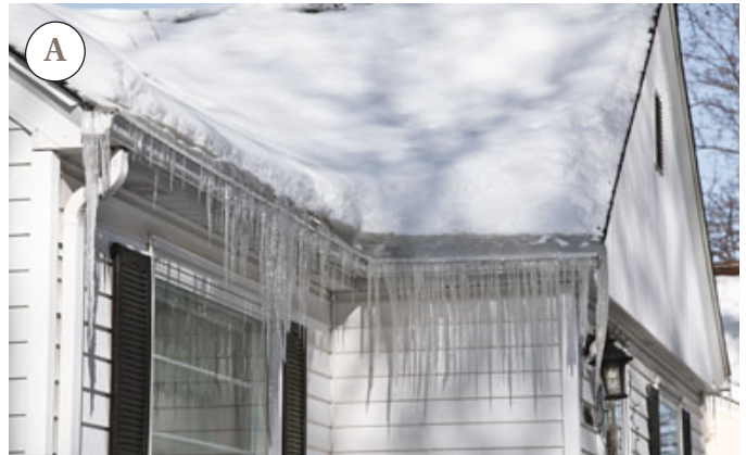
Figure 2. Ice dams form on cold days when heat leaking from inside the home warms the attic enough to melt the snow on the roof (A). Damaging leaks may show up in subtle ways, like this line of ice emanating from behind the siding (B), or not so subtly, in the case of icicles growing out of a soffit (C). Tannin stains on the siding of this home (D) are unmistakable evidence that lumber in the structure is being drenched with snowmelt.
