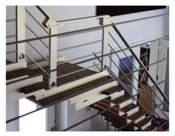
Modular Stairs. Instead of a one-piece stringer, an *Ascendings* modular staircase has individual CNC-machined aluminum "risers." Since the risers and treads
