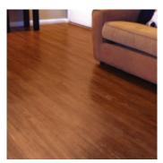
to wear and tear better than competing vinyl flooring. Installation requires tile adhesive and a 100-pound roller. Planks cost about \$1 per square foot and tiles \$1.20 per square foot.
