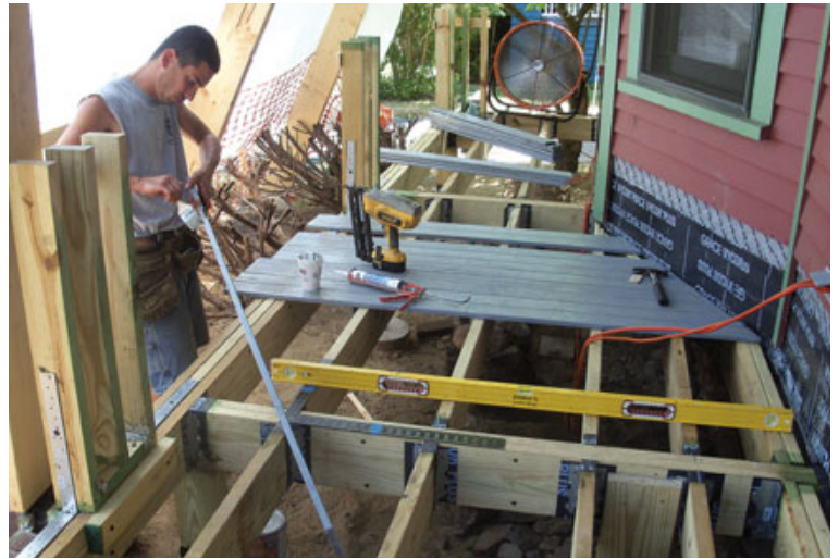
Figure 2. With the deck framing resting on temporary supports, the author lays out and installs the post anchors (left), ensuring accurate positioning of the pressure-treated 6x6s (below left). Short sections of knee wall were attached to the front of the deck with metal straps and framing anchors; later they would be enclosed by finished PVC pillars (below).
