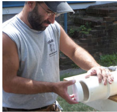
Figure 6. A carbide blade in a circular saw was used to trim the bottom ends of the columns to length (left). The tops were trickier: In order to exactly match the original columns, the author had to add a few inches to the top. He did this by inserting a PVC plug (center) — which he screwed in place inside the column, flush with the top — and then adding PVC extension pieces, which he screwed to the plug (right).
