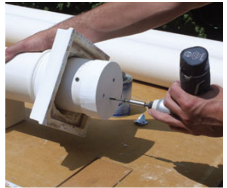
Figure 6. A carbide blade in a circular saw was used to trim the bottom ends of the columns to length (left). The tops were trickier: In order to exactly match the original columns, the author had to add a few inches to the top. He did this by inserting a PVC plug (center) — which he screwed in place inside the column, flush with the top — and then adding PVC extension pieces, which he screwed to the plug (right).
