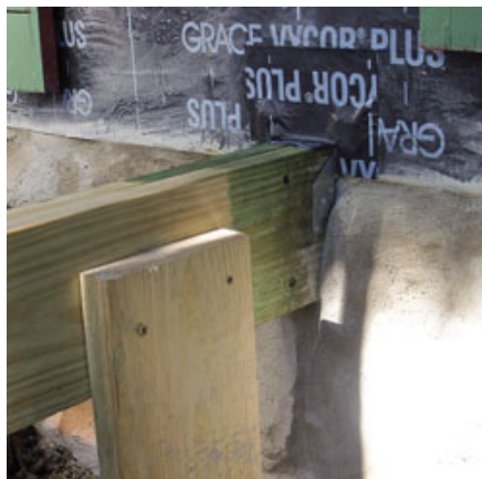
Figure 1. Rotted girders in the old framing (above left) extended just an inch into poorly hewn pockets in the rough stone foundation. The author repointed and parged the existing pockets and cut additional ones for new double 2x10 beams. Cut ends of the pressure-treated lumber were soaked with wood preservative, and metal hangers were added for an extra measure of stability (above). Peel-and-stick membrane protects the hardware and seals the beam pocket (left).
