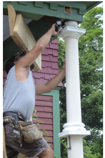
Figure 7. Metal framing anchors screwed to the column (above left) provide a strong connection to the pedestal. The tops are secured with screws angled into the roof girder (above). At left, the finished colonnade.
