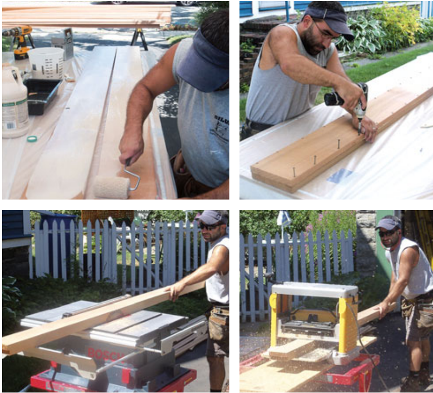
Figure 4. Thick handrail and baluster stock was laminated from 5/4 red cedar. The boards were glued (top left) and screwed (top right) together. After the glue had set overnight, the built-up stock was ripped to width and thickness-planed (above left and right).
