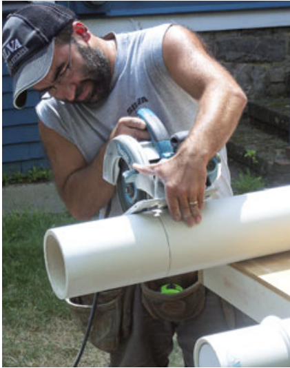
Figure 6. A carbide blade in a circular saw was used to trim the bottom ends of the columns to length (left). The tops were trickier: In order to exactly match the original columns, the author had to add a few inches to the top. He did this by inserting a PVC plug (center) — which he screwed in place inside the column, flush with the top — and then adding PVC extension pieces, which he screwed to the plug (right).
