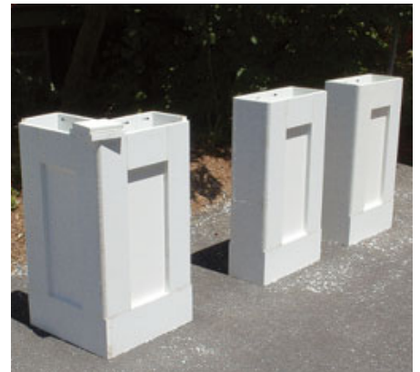
Figure 3. The author used pocket screws (above left) and cement to assemble the frames of the cellular PVC pedestals (above). The completed pedestals were slipped in place over the framed knee walls, then trimmed with PVC moldings to hide fastener holes (left).
