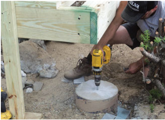
Figure 2. With the deck framing resting on temporary supports, the author lays out and installs the post anchors (left), ensuring accurate positioning of the pressure-treated 6x6s (below left). Short sections of knee wall were attached to the front of the deck with metal straps and framing anchors; later they would be enclosed by finished PVC pillars (below).
