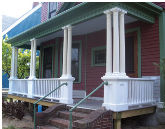
Figure 7. Metal framing anchors screwed to the column (above left) provide a strong connection to the pedestal. The tops are secured with screws angled into the roof girder (above). At left, the finished colonnade.
