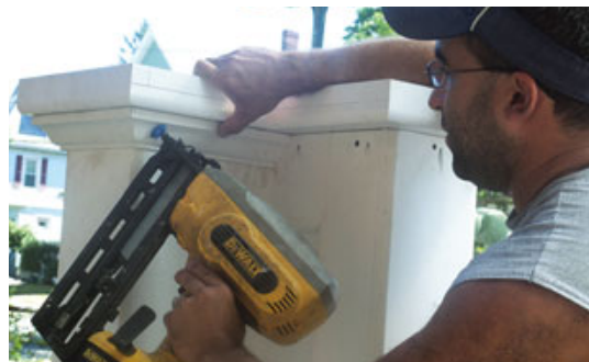
Figure 3. The author used pocket screws (above left) and cement to assemble the frames of the cellular PVC pedestals (above). The completed pedestals were slipped in place over the framed knee walls, then trimmed with PVC moldings to hide fastener holes (left).
