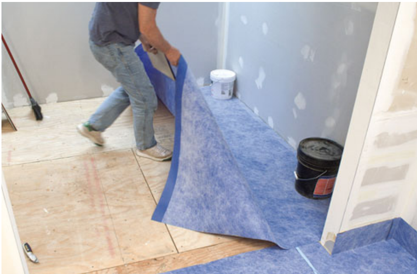
Figure 7. To speed up sheet membrane installation, the author cuts, dry-fits, and folds all sections before applying adhesive. First, he positions the cut sheet (top), secures the back of the sheet with weighted buckets, and lifts it out of the way (above). He folds the loose end back, weighing it down with tiles (right) while he prepares to spread adhesive.
