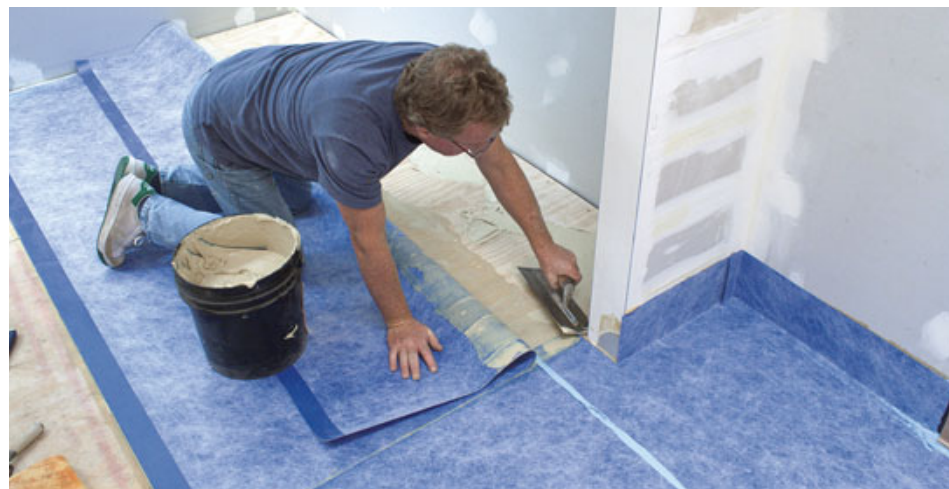
Figure 8. When the contact cement becomes tacky (which takes about 10 to 20 minutes), the author unfolds the loose end of the membrane (top) and laminates the sheet with a straightedge (above). With the front of the sheet laminated, he pulls the back portion forward and spreads contact cement for the rest of the sheet (left).
