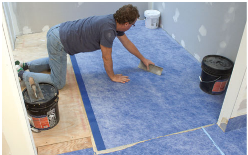
Figure 8. When the contact cement becomes tacky (which takes about 10 to 20 minutes), the author unfolds the loose end of the membrane (top) and laminates the sheet with a straightedge (above). With the front of the sheet laminated, he pulls the back portion forward and spreads contact cement for the rest of the sheet (left).
