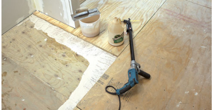
Figure 4. The plywood underlayment is partially installed. Note that glue was spread a few inches beyond the footprint of the plywood sheets. As subsequent boards are secured, any exposed glue not covered within five minutes or so should be removed with a scraper and damp sponge.
