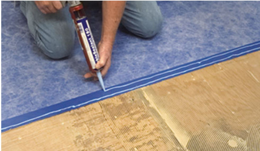
Figure 9. For a flat and leakproof seam in the sheet membrane, the author lays down two beads of manufacturer-supplied sealant (above) and flattens the seam with a straightedge (left). Sealant squeeze-out indicates the seam is closed.
