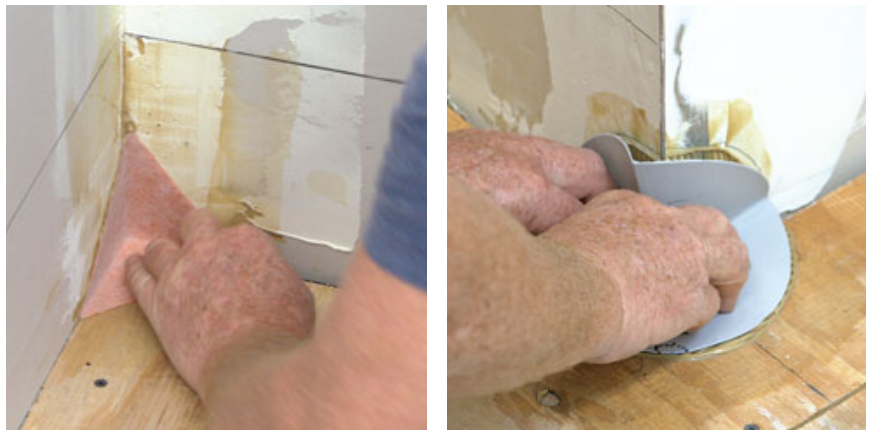
Figure 6. For maximum waterproofing protection, the author installs factory-made accessories like these corner pieces. He works the inside corner (left) and outside corner pieces (right) into the contact cement with his fingers.
