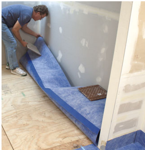
Figure 7. To speed up sheet membrane installation, the author cuts, dry-fits, and folds all sections before applying adhesive. First, he positions the cut sheet (top), secures the back of the sheet with weighted buckets, and lifts it out of the way (above). He folds the loose end back, weighing it down with tiles (right) while he prepares to spread adhesive.
