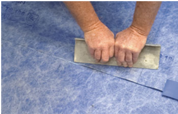
Figure 9. For a flat and leakproof seam in the sheet membrane, the author lays down two beads of manufacturer-supplied sealant (above) and flattens the seam with a straightedge (left). Sealant squeeze-out indicates the seam is closed.
