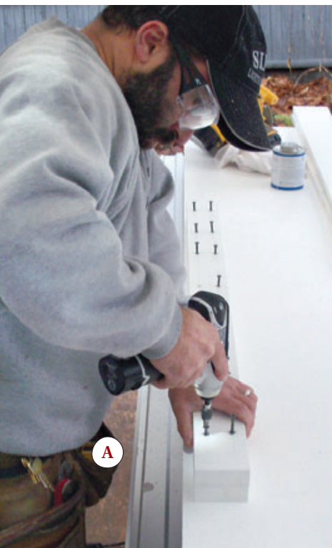
Figure 9. The exterior sill is built up from two thicknesses of material fastened with cement and screws; the screws are spaced back from the edges to avoid contact with the saw blade when the stock is ripped to the required angle (A, B). The countersunk screw holes are filled with manufactured plugs and cut flush (C).
