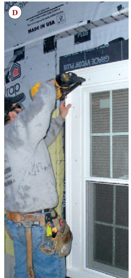
Figure 11. Once the trim unit has been tacked in place and leveled, the screws are driven home, starting at the bottom (A, B). A PVC trim band covers the outer row of screws (C, D); the remaining holes are plugged.
