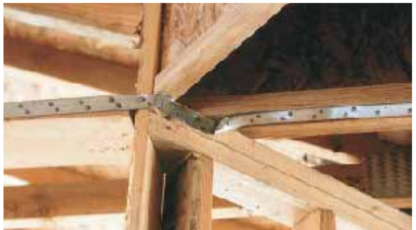
Figure 12. Straps should not be bent: The kink in this strap weakens it.
