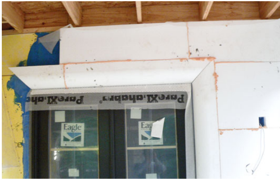
Figure 3. The author fabricates trim details like these bullnose returns (left) with a hot wire cutter. After the foam has been glued to the walls, all of the gaps between panels are filled with spray foam (above).
