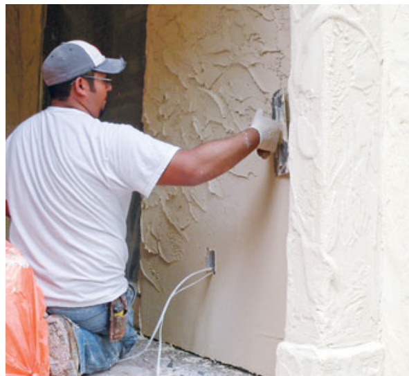
Figure 5. Most EIF systems have a smooth and uniform finish coat, but this home was given a deeply textured finish coat to match the Mediterranean architecture.
