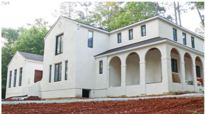
Figure 7. Corbels and other architectural details can be added to EIFS cladding by gluing foam profiles to the EPS before applying the base coat and finish. Areas that don't require insulation, like the columns supporting the arches on this home, can be wrapped with cement backerboard instead of foam, which gives them better impact resistance.
