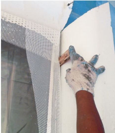
Figure 3. The author fabricates trim details like these bullnose returns (left) with a hot wire cutter. After the foam has been glued to the walls, all of the gaps between panels are filled with spray foam (above).
