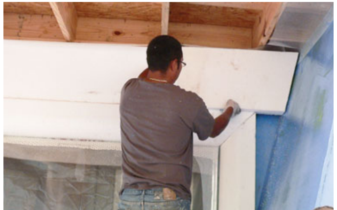
Figure 2. Once the WeatherSeal membrane has been installed, DrainEdge termination strips are stapled over door and window openings, followed by back-wrapping mesh (above). The EPS panels are glued to the walls with adhesive that's been applied with a notched trowel (above right, right). The notches are vertically oriented so that moisture can drain down the channels between the membrane and the foam and out of the wall assembly wherever the DrainEdge has been installed.
