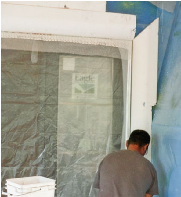
Figure 2. Once the WeatherSeal membrane has been installed, DrainEdge termination strips are stapled over door and window openings, followed by back-wrapping mesh (above). The EPS panels are glued to the walls with adhesive that's been applied with a notched trowel (above right, right). The notches are vertically oriented so that moisture can drain down the channels between the membrane and the foam and out of the wall assembly wherever the DrainEdge has been installed.
