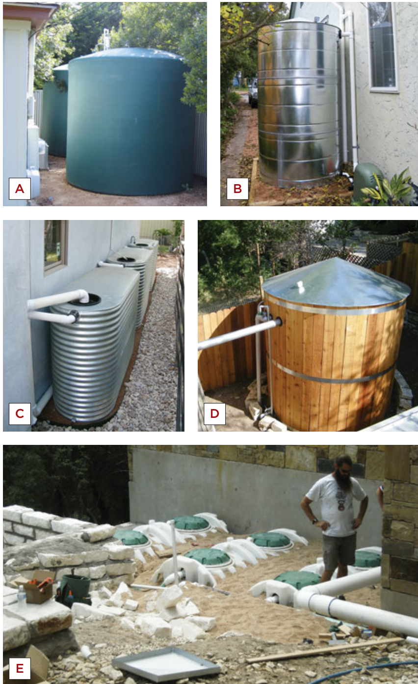
Figure 5. Tucked away behind the garage, these two plastic tanks (A) provide 6,000 gallons of storage. Custom-fabricated steel tanks (B) are more attractive, so there is less need to hide them away. Some tanks are designed to fit an available space — under a deck, say, or in a narrow side yard (C). Because there was no place to hide it in an urban lot, this plastic tank (D) was clad with cedar and given a metal top. Some tanks (E) are designed to be buried and thus kept out of sight.
