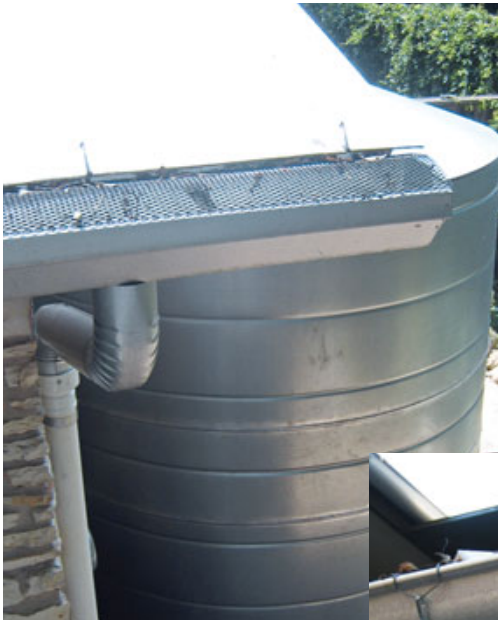
Figure 3. Solid debris such as leaves and twigs are kept out of the system by screening the tops of the gutters (above) and installing a rain head (right) in the downspout. The sloped screen of the rain head diverts debris into the yard while allowing water to pass through. A second, finer screen underneath prevents mosquitoes and other insects from getting into the tank.
