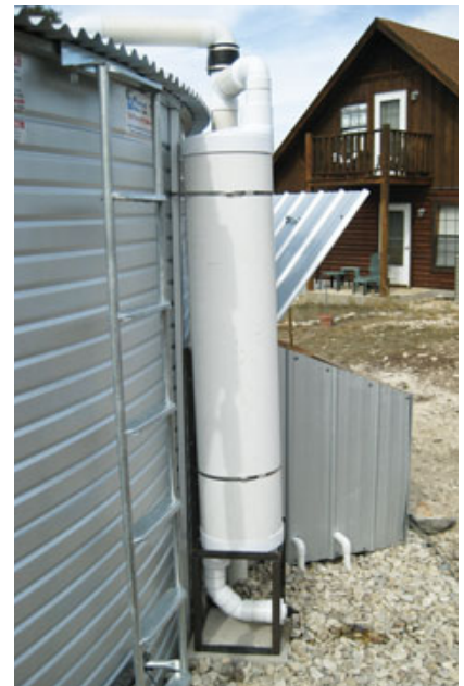
Figure 4. A first-flush diverter keeps dissolved dirt and bird droppings from getting into the tank. It does this by discarding the first water that flows off the roof in a storm, diverting it to a chamber that slowly drains onto the ground. The diverter kit includes everything except the pipe for the diversion chamber, which is sized by the installer based on roof area. Shown here are a small diverter pipe for a single-tank dry-pipe system (photo, top right) and a large diverter chamber on a wet-pipe potable system (photo, right).
