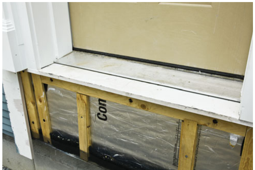
Figure 2. To provide an unobstructed swing, exterior doors were installed as if in a conventional 2x6 wall (left). Exterior extensions to the jambs and threshold rely on composite lumber and caulk (below).
