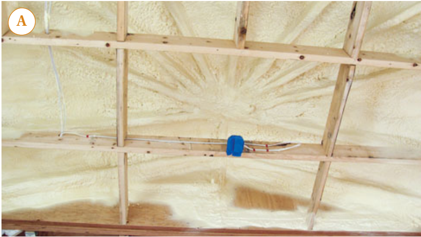
Figure 6. Complex framing areas are ideal spray-foam candidates (A). At roughly R-6 per inch, the 2x8 framing bays approach a nominal R-44. Two doghouse dormers were also insulated with closed-cell foam (B). The finished basement walls were insulated to R-25 with a combination of 2-inch XPS foam and R-15 fiberglass batts (C). Note the air-sealing tape over the seams. Spray foam on the rim joist laps onto the XPS on the foundation walls, creating an air seal along the top of the board (D).
