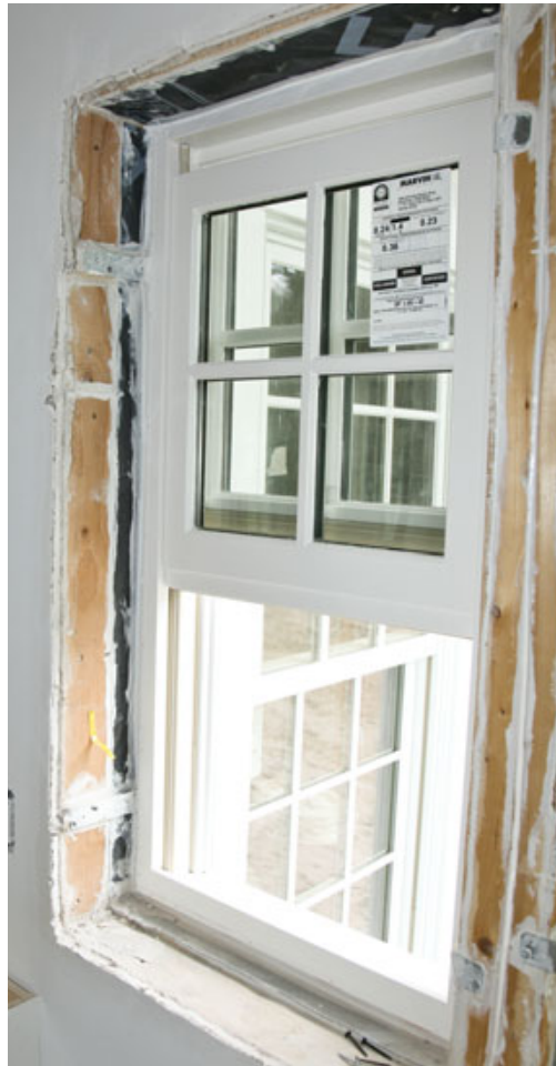
Figure 7. Leaving little to chance, the crew caulked all seams between framing members and subfloor (top). Foam backer rod, sealed with caulk, was used in lieu of expanding foam around window and door jambs (above). Window sealing was time-consuming, with caulk outlining the metal installation straps and the interior edges of the self-adhering window flashing (right).
