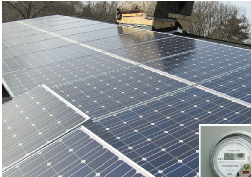
Figure 10. A 7-kW PV array on the shed-dormer roof is projected to supply more than 100 percent of the home's electrical consumption (above). A digital electric meter displays a constant readout of power delivered to and from the grid (right).
