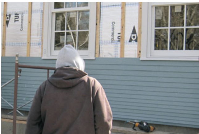
Figure 4. The fiber-cement siding was custom-ripped to allow narrower courses and tighter stacking at the base of the wall.
