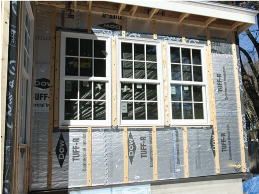
Figure 3. The sheathing is strapped on 2-foot centers, directly over the wall framing (left). The top of the venting channels is open to the soffit, ensuring positive airflow from the bottom up. Ridge-vent material blocks the gaps between strapping, forcing an insect barrier screen against the back of the siding (above).
