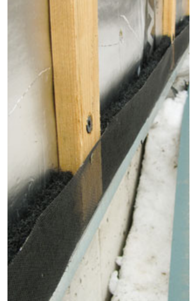
Figure 3. The sheathing is strapped on 2-foot centers, directly over the wall framing (left). The top of the venting channels is open to the soffit, ensuring positive airflow from the bottom up. Ridge-vent material blocks the gaps between strapping, forcing an insect barrier screen against the back of the siding (above).
