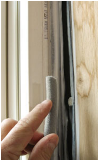
Figure 7. Leaving little to chance, the crew caulked all seams between framing members and subfloor (top). Foam backer rod, sealed with caulk, was used in lieu of expanding foam around window and door jambs (above). Window sealing was time-consuming, with caulk outlining the metal installation straps and the interior edges of the self-adhering window flashing (right).
