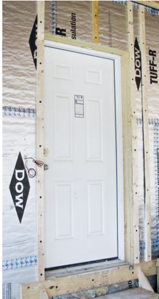
Figure 2. To provide an unobstructed swing, exterior doors were installed as if in a conventional 2x6 wall (left). Exterior extensions to the jambs and threshold rely on composite lumber and caulk (below).
