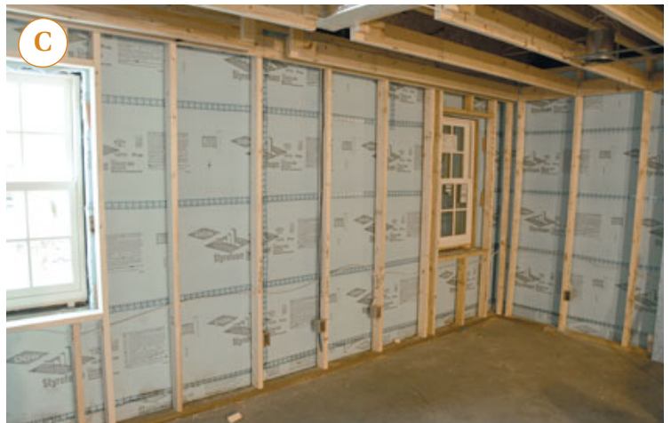
Figure 6. Complex framing areas are ideal spray-foam candidates (A). At roughly R-6 per inch, the 2x8 framing bays approach a nominal R-44. Two doghouse dormers were also insulated with closed-cell foam (B). The finished basement walls were insulated to R-25 with a combination of 2-inch XPS foam and R-15 fiberglass batts (C). Note the air-sealing tape over the seams. Spray foam on the rim joist laps onto the XPS on the foundation walls, creating an air seal along the top of the board (D).
