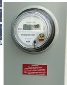
Figure 10. A 7-kW PV array on the shed-dormer roof is projected to supply more than 100 percent of the home's electrical consumption (above). A digital electric meter displays a constant readout of power delivered to and from the grid (right).
