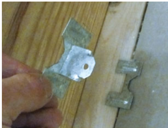
Figure 9. Drywall clips replace lumber backers in wall and ceiling corners.
