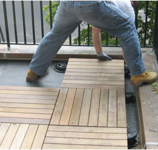
Figure 5. To prevent lateral shifting, a maximum clearance of \frac{1}{4} inch is allowed around the deck's perimeter. The author installed an ipe border in the gap between the parapet and field tiles (above), supported between pedestals with custom-made ipe biscuits (right).
