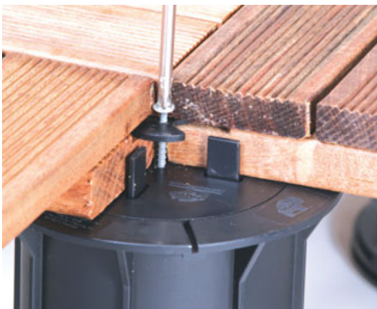
Figure 4. A plastic disk and a single screw secure the corners of four ipe tiles at every pedestal (above). Spacer tabs maintain a uniform 1/4 -inch gap between adjacent tiles; a wedge-shaped cutout in the disk can be rotated to allow a tile to be removed. Tiles and pedestals are installed and leveled one at a time (right).
