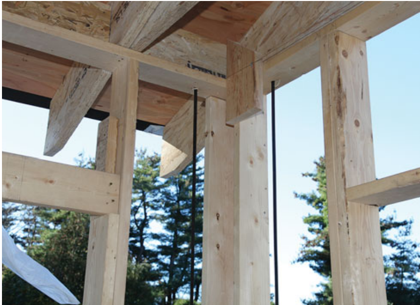
Figure 3. Intermittent vertical 4-by-10-foot sheets of 1/2-inch CDX plywood applied directly to the frame brace it against wind racking (top). Hold-down rods — required with intermittent bracing — are installed at building corners and at regular intervals around the perimeter. They're anchored in the foundation and continue up the walls (above) through the topmost wall plate (left).
