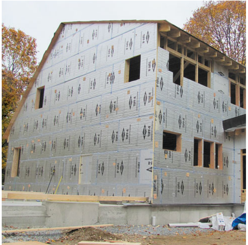
Figure 5. Before framing the unheated attached garage, the author applied foam sheathing to the common wall, establishing a thermal break between the two structures (above). Structural screws driven through the foam tie the isolated frames together. Here, the author anchors a walk-out bay rafter to the wall framing (left).
