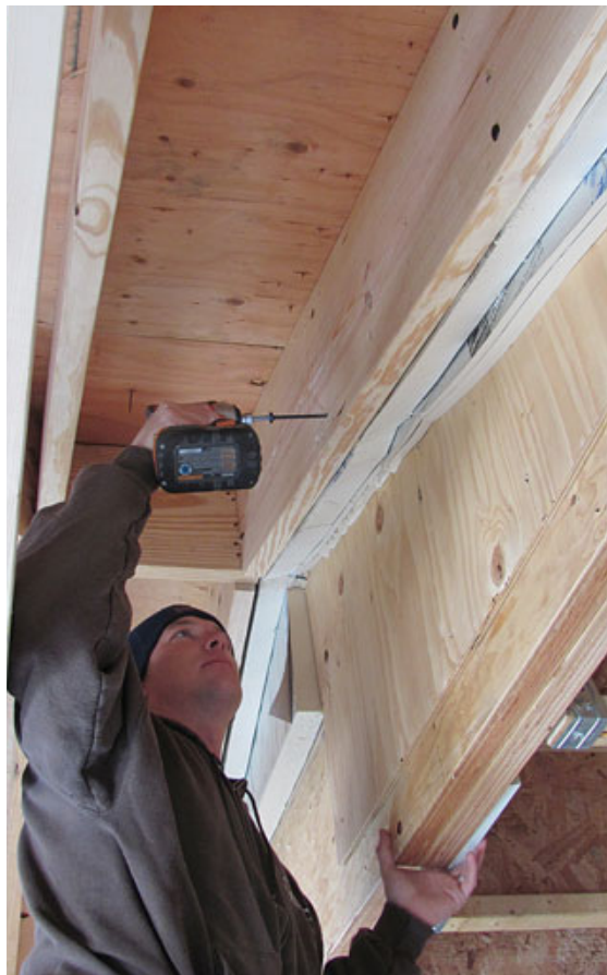
Figure 5. Before framing the unheated attached garage, the author applied foam sheathing to the common wall, establishing a thermal break between the two structures (above). Structural screws driven through the foam tie the isolated frames together. Here, the author anchors a walk-out bay rafter to the wall framing (left).
