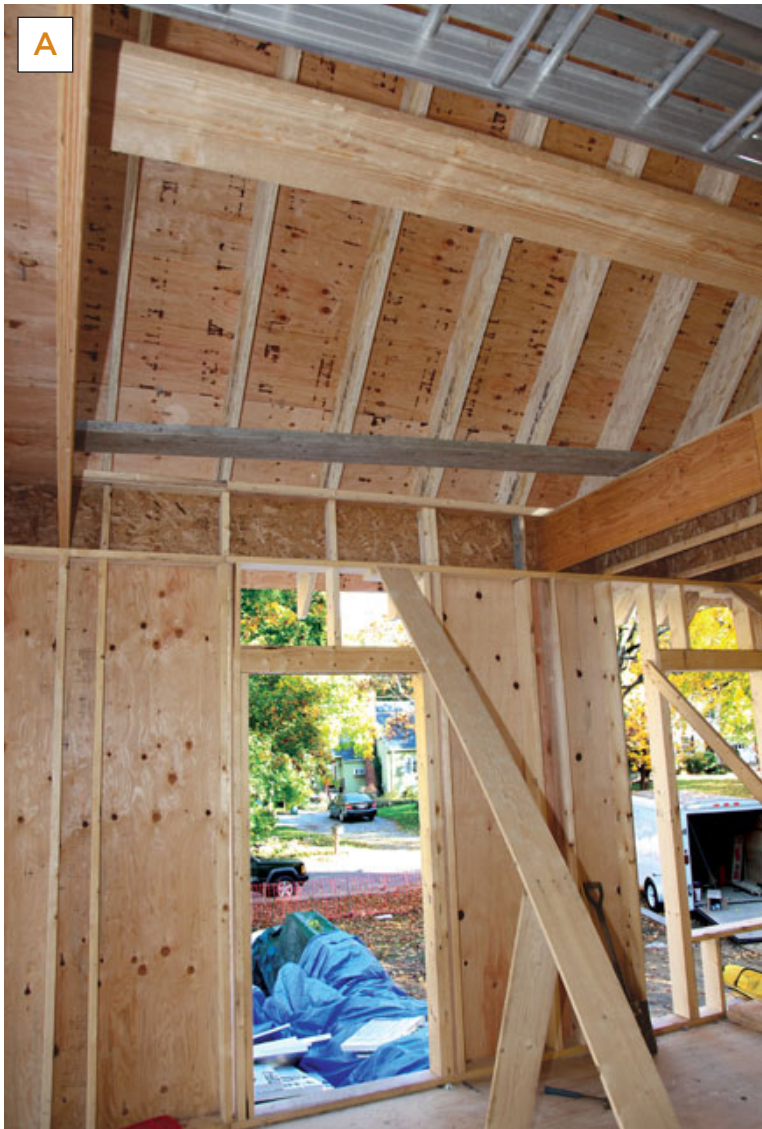
Figure 1. In an advanced frame, headers are minimized in favor of insulation cavities. All framing is vertically aligned and point loads are distributed directly through to the foundation. In this sloped ceiling section, squash blocks carry the rafters' load path over the second-floor rim joist (A). Where interior partitions intersect exterior walls, horizontal ladder blocking will secure the end stud, keeping the wall bay fully open and accessible for insulation (B). Structural headers are packed with foam board to create a thermal break (C). Openings in nonbearing walls are minimally framed, with single-member headers installed on the flat (D). The 1/2-inch plywood lining the rough opening extends out to cap the edge of the 4-inch-thick foam sheathing.
