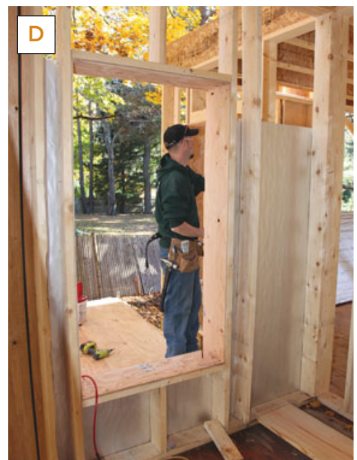
Figure 1. In an advanced frame, headers are minimized in favor of insulation cavities. All framing is vertically aligned and point loads are distributed directly through to the foundation. In this sloped ceiling section, squash blocks carry the rafters' load path over the second-floor rim joist (A). Where interior partitions intersect exterior walls, horizontal ladder blocking will secure the end stud, keeping the wall bay fully open and accessible for insulation (B). Structural headers are packed with foam board to create a thermal break (C). Openings in nonbearing walls are minimally framed, with single-member headers installed on the flat (D). The 1/2-inch plywood lining the rough opening extends out to cap the edge of the 4-inch-thick foam sheathing.
