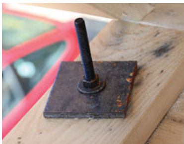
Figure 3. Intermittent vertical 4-by-10-foot sheets of 1/2-inch CDX plywood applied directly to the frame brace it against wind racking (top). Hold-down rods — required with intermittent bracing — are installed at building corners and at regular intervals around the perimeter. They're anchored in the foundation and continue up the walls (above) through the topmost wall plate (left).
