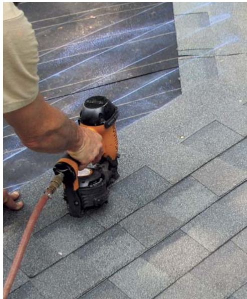
Figure 8. The “Tamko” valley is a fast, watertight, manufacturer-approved method for completing a valley, but it’s best-suited to laminated shingles, where its sawtooth pattern remains inconspicuous. One slope — the shallower, if applicable — is completed first, with its courses running across the valley by at least 12 inches. To outline the valley, whole shingles are then nailed end-to-end along a chalk line. An optional bead of roofing mastic adds insurance against uplift (left). The opposite slope is completed from the valley line back, with square-cut corners toeing the valley line (center). A dab of mastic glues the sawtooth tips to the valley starter (right).
