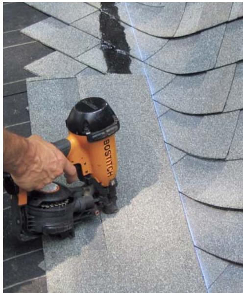
Figure 8. The “Tamko” valley is a fast, watertight, manufacturer-approved method for completing a valley, but it’s best-suited to laminated shingles, where its sawtooth pattern remains inconspicuous. One slope — the shallower, if applicable — is completed first, with its courses running across the valley by at least 12 inches. To outline the valley, whole shingles are then nailed end-to-end along a chalk line. An optional bead of roofing mastic adds insurance against uplift (left). The opposite slope is completed from the valley line back, with square-cut corners toeing the valley line (center). A dab of mastic glues the sawtooth tips to the valley starter (right).
