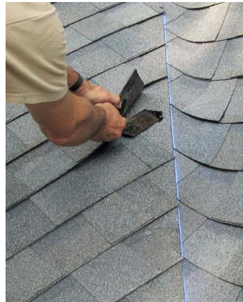
Figure 8. The “Tamko” valley is a fast, watertight, manufacturer-approved method for completing a valley, but it’s best-suited to laminated shingles, where its sawtooth pattern remains inconspicuous. One slope — the shallower, if applicable — is completed first, with its courses running across the valley by at least 12 inches. To outline the valley, whole shingles are then nailed end-to-end along a chalk line. An optional bead of roofing mastic adds insurance against uplift (left). The opposite slope is completed from the valley line back, with square-cut corners toeing the valley line (center). A dab of mastic glues the sawtooth tips to the valley starter (right).
