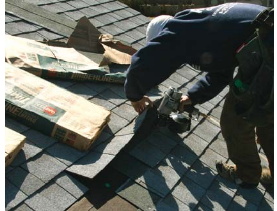
Figure 6. Chalk lines are measured against the ridge line to ensure a parallel outcome. Here, the line guides the layout beyond a completed open valley and provides alignment for the opposite slope (left). Shingles are initially nailed high, then secured in the fastening zone to complete the infill (above).
