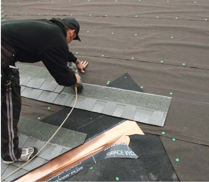
Figure 6. Chalk lines are measured against the ridge line to ensure a parallel outcome. Here, the line guides the layout beyond a completed open valley and provides alignment for the opposite slope (left). Shingles are initially nailed high, then secured in the fastening zone to complete the infill (above).
