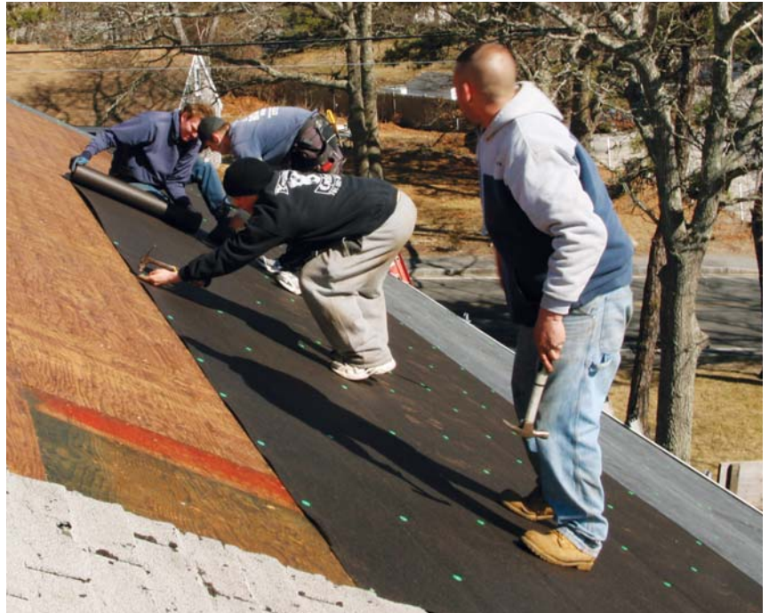
Figure 2. Carefully installed underlayment is the last best defense against ice dams and wind-driven rain (above). Plastic caps (left) provide superior holding power and prevent the roofing paper from tearing around fasteners. Slopes from 4/12 to 2/12 are covered with self-adhering membrane, which is also run up the rakes to protect the trim.
