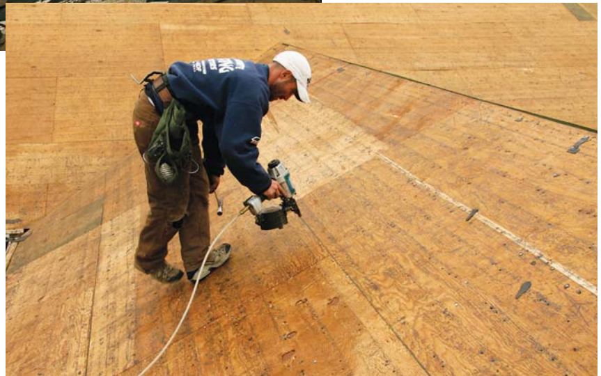
Figure 1. Stripping the roof down to the sheathing exposes any hidden problems and provides the best conditions for reinstallation (left). The author strongly advises renauling afterward because stripping shingles can loosen sheathing nails. Workers carry a hammer along with the nail gun to whack down stray nail heads (below).
