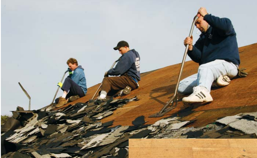
Figure 1. Stripping the roof down to the sheathing exposes any hidden problems and provides the best conditions for reinstallation (left). The author strongly advises renauling afterward because stripping shingles can loosen sheathing nails. Workers carry a hammer along with the nail gun to whack down stray nail heads (below).
