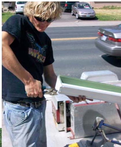
Figure 2. Besides the gutter machine, the author's tools are mostly simple hand tools (above left), including a snap-lock punch for attaching end caps (above) and a gutter outlet punch for making clean downspout holes (left).
