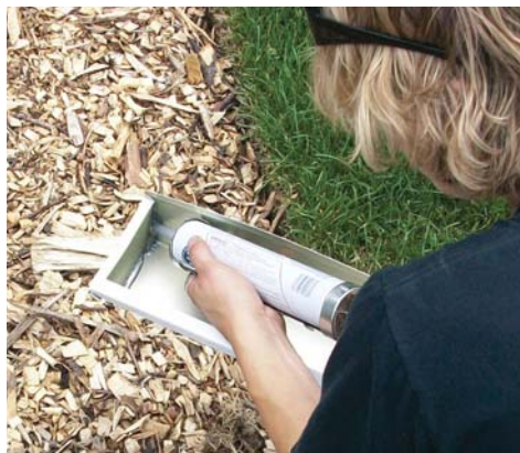
Figure 4. The author uses Ruscoe 12-1 Seam Sealer, which is specifically designed for gutter work. It flows and seals better than conventional caulks.
