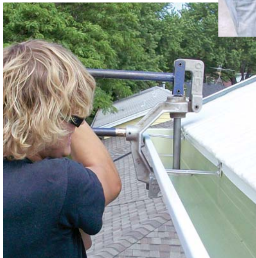
Figure 2. Besides the gutter machine, the author's tools are mostly simple hand tools (above left), including a snap-lock punch for attaching end caps (above) and a gutter outlet punch for making clean downspout holes (left).
