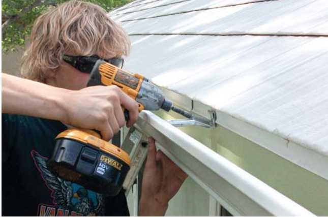
Figure 6. Forget gutter spikes: Fascia hangers with the fastening screw already in place speed the job and provide great support.
