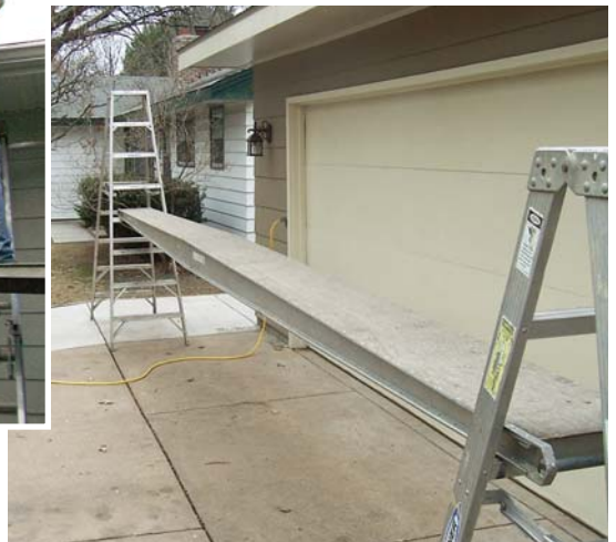
Figure 3. Staging for gutter jobs must be placed far enough out from the house to allow the crew to work safely at the outer edge of the roof overhang.
