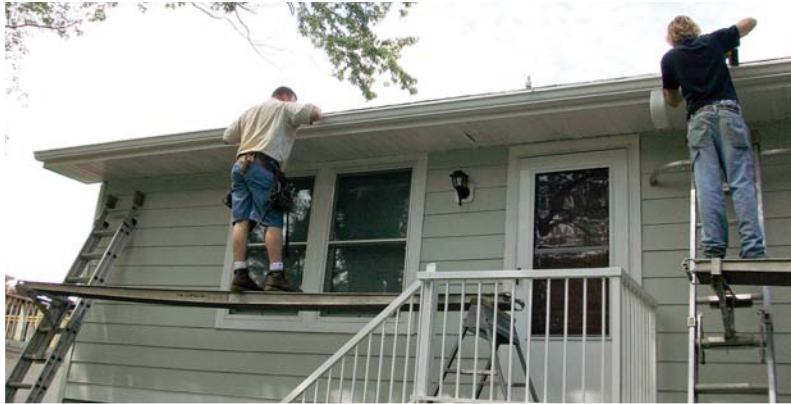
Figure 3. Staging for gutter jobs must be placed far enough out from the house to allow the crew to work safely at the outer edge of the roof overhang.
