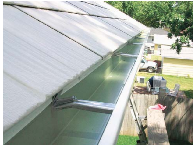
Figure 6. Forget gutter spikes: Fascia hangers with the fastening screw already in place speed the job and provide great support.
