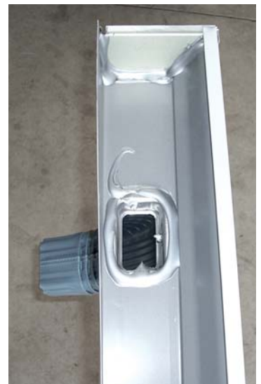
Figure 4. The author uses Ruscoe 12-1 Seam Sealer, which is specifically designed for gutter work. It flows and seals better than conventional caulks.
