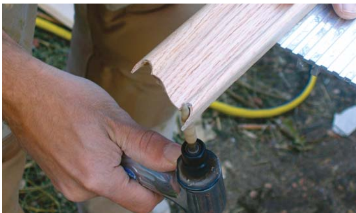
Figure 4. The author uses a die-grinder to cope the 180-degree curves on cap molding (above) and to preserve the more delicate parts of a one-piece baseboard (right). He copes the straight part of the baseboard by making a stopped cut with a miter saw.
