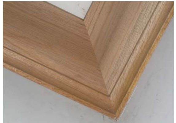
Figure 5. Normally the small projection at the bottom of this crown (far left) would be cut off, but instead the author makes a 45-degree notch in the edge of the adjoining piece (left). When the pieces are installed, the cope fits perfectly and — viewed from below — looks like a miter (below).
