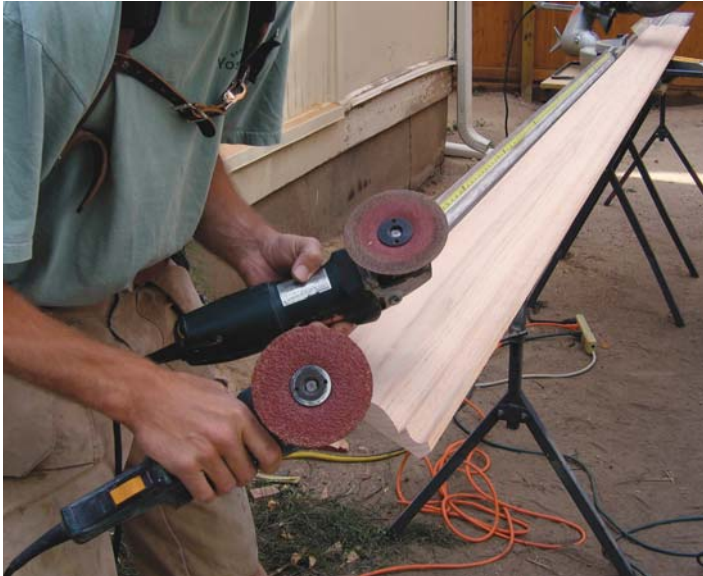
Figure 1. Instead of switching disks, the author switches grinders: He puts 24-grit paper on one tool and uses it for fast stock removal, and 50-grit on the other for precise finishing cuts (left). Curves too tight to grind with a disk are cut with a die grinder equipped with a tapered carbide carving burr or a cone-shaped metalworking burr (above).
