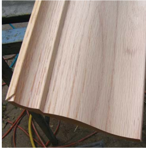
Figure 5. Normally the small projection at the bottom of this crown (far left) would be cut off, but instead the author makes a 45-degree notch in the edge of the adjoining piece (left). When the pieces are installed, the cope fits perfectly and — viewed from below — looks like a miter (below).
