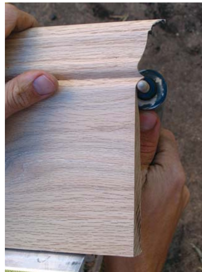
Figure 4. The author uses a die-grinder to cope the 180-degree curves on cap molding (above) and to preserve the more delicate parts of a one-piece baseboard (right). He copes the straight part of the baseboard by making a stopped cut with a miter saw.
