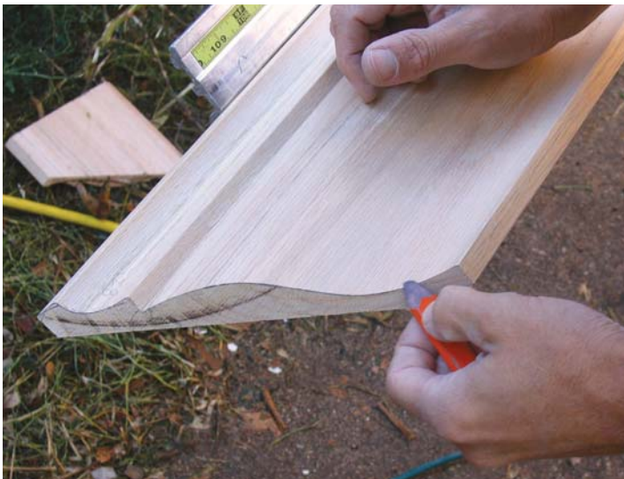
Figure 2. Highlighting the cope line with a pencil makes it easier to see.
