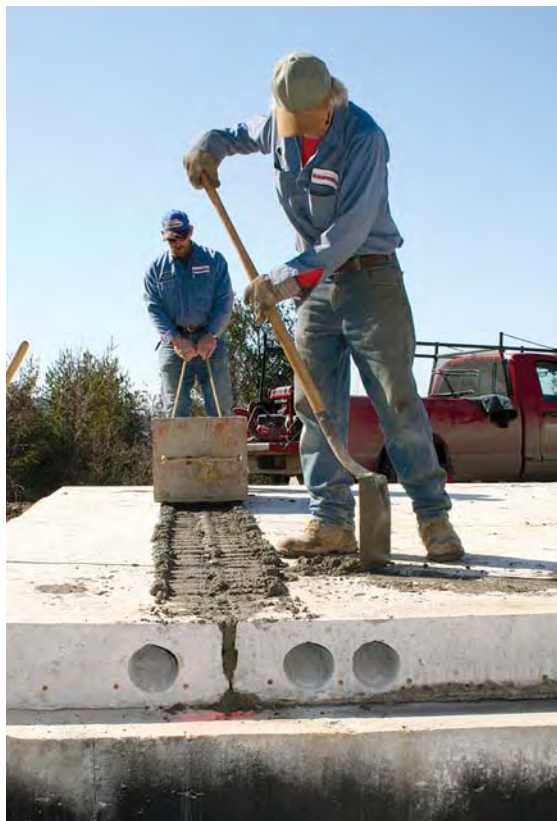
Figure 4. Keyways between planks are fitted with backer rod (above), then filled with high-strength nonshrink cement grout (left).
