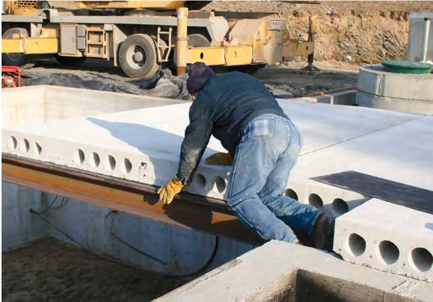
Figure 3. When there is an opening in the floor system, planks can be supported by steel beams (above) or by special steel brackets supplied by the fabricator (right); plastic shims are used to help level the planks. Where the planks bear on the foundation walls, steel plates cast into both the planks and the foundation are welded together (below right).
