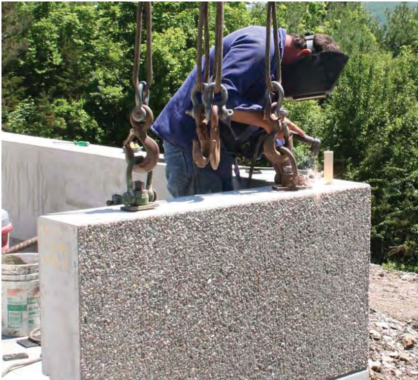
Figure 7. After assembly, the metal corner connector plates (top photos) are welded together (above). Once the panels are in place (right), regular framing and door and window installation can begin.
