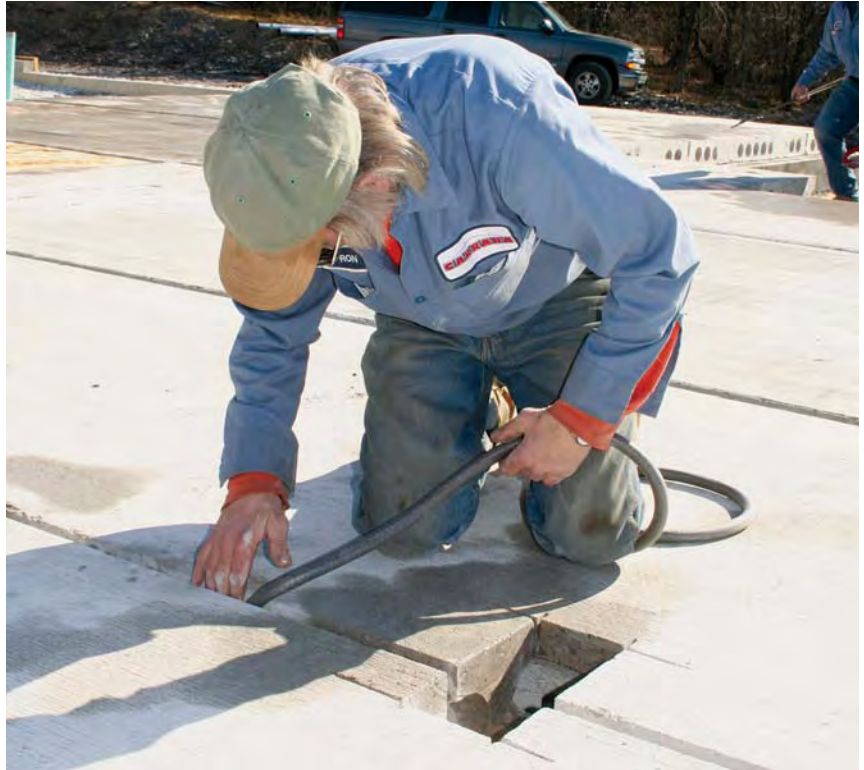
Figure 4. Keyways between planks are fitted with backer rod (above), then filled with high-strength nonshrink cement grout (left).
