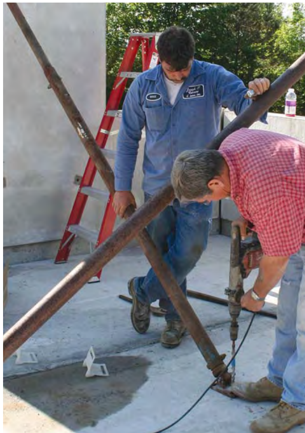
Figure 6. Rebar pins at the base of each wall panel slide into holes bored into the top of the foundation wall (above); the holes are filled with grout before installation, and plastic shims are used to level the panels. Braces lock the panels into position until the framing is completed (left).
