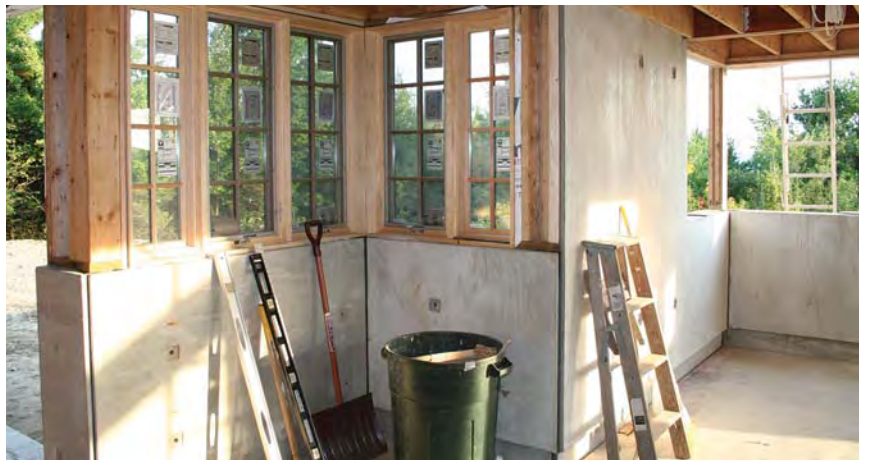
Figure 7. After assembly, the metal corner connector plates (top photos) are welded together (above). Once the panels are in place (right), regular framing and door and window installation can begin.
