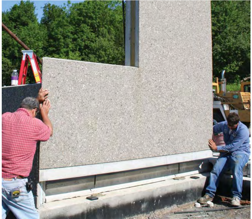
Figure 6. Rebar pins at the base of each wall panel slide into holes bored into the top of the foundation wall (above); the holes are filled with grout before installation, and plastic shims are used to level the panels. Braces lock the panels into position until the framing is completed (left).
