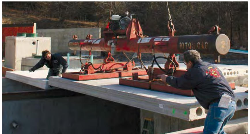
Figure 1. Hollow-core planks are slip-cast on long beds, tensioned with wire strand, then cut to length after the concrete has cured (top). The planks are cambered but will flatten out when loaded — with a 3-inch topping slab, in the case shown here (above). A crane is needed to maneuver the 8-foot-wide planks on the job site (right).
