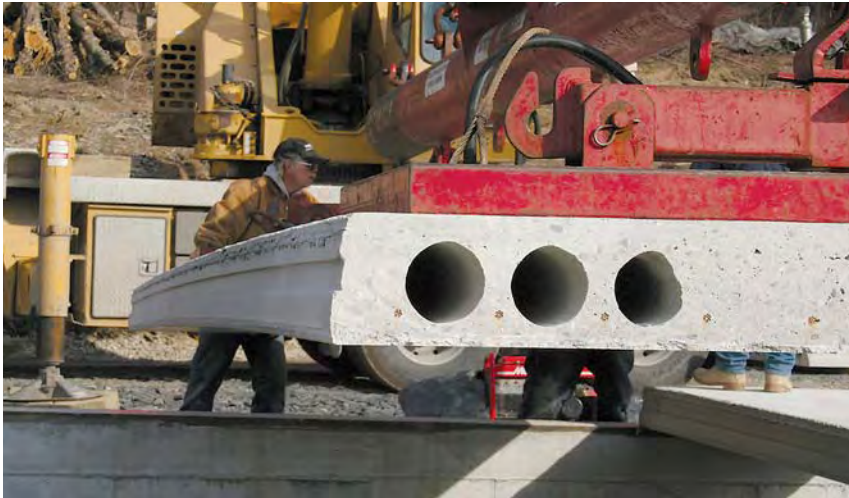
Figure 1. Hollow-core planks are slip-cast on long beds, tensioned with wire strand, then cut to length after the concrete has cured (top). The planks are cambered but will flatten out when loaded — with a 3-inch topping slab, in the case shown here (above). A crane is needed to maneuver the 8-foot-wide planks on the job site (right).
