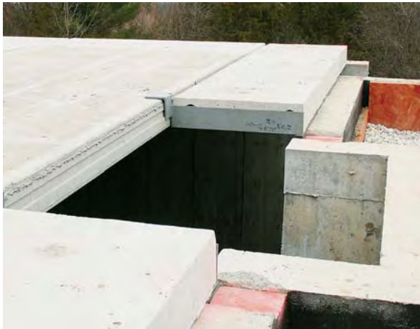
Figure 3. When there is an opening in the floor system, planks can be supported by steel beams (above) or by special steel brackets supplied by the fabricator (right); plastic shims are used to help level the planks. Where the planks bear on the foundation walls, steel plates cast into both the planks and the foundation are welded together (below right).
