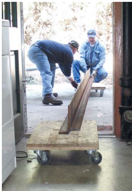
Figure 3. At about 200 pounds each, the T-shaped pieces of steel were light by structural steel standards. A pair of four-wheel dollies (above) and a drywall lift (right) made the job easier.
