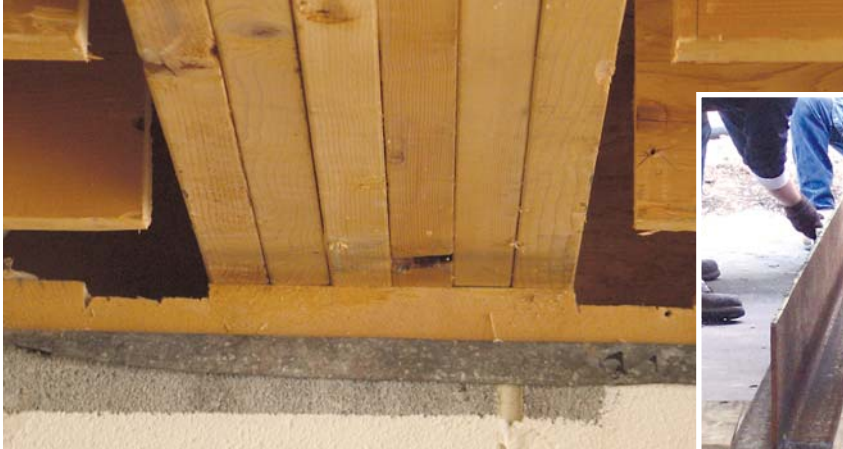
Figure 4. The mudsill was notched (above) so the joist ends would rest on the top of the outer flange of each WT beam (right). Since removing material from under the existing girder would have been difficult, one side of the WT flanges was cut away instead (inset).
