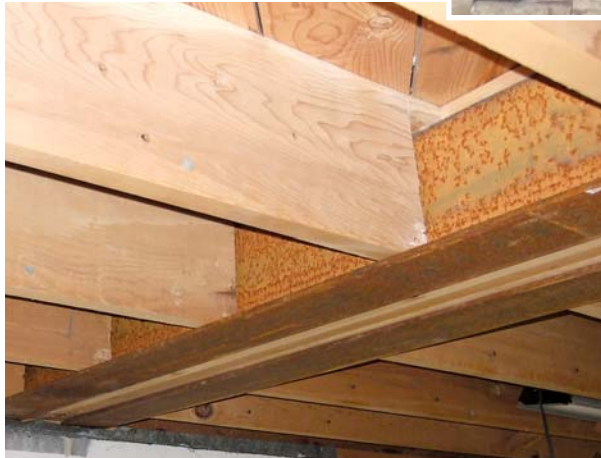
Figure 4. The mudsill was notched (above) so the joist ends would rest on the top of the outer flange of each WT beam (right). Since removing material from under the existing girder would have been difficult, one side of the WT flanges was cut away instead (inset).
