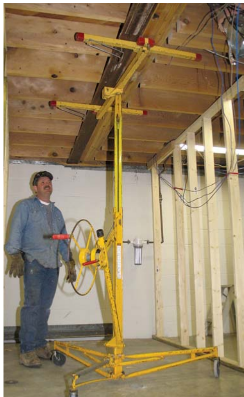
Figure 3. At about 200 pounds each, the T-shaped pieces of steel were light by structural steel standards. A pair of four-wheel dollies (above) and a drywall lift (right) made the job easier.
