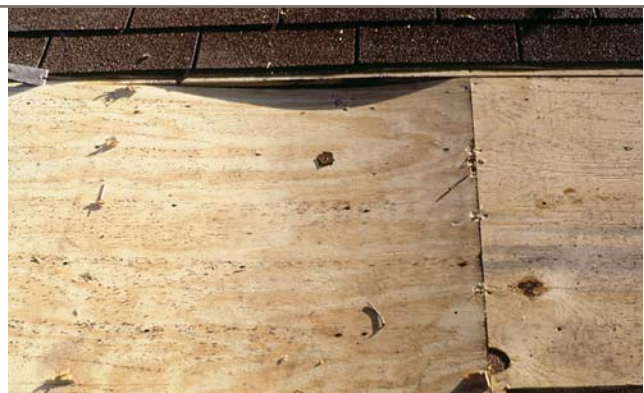
The use of self-spacing H-clips would have prevented this roof sheathing from buckling, which can occur either along the edge (above) or at the end (left) of panels that have been installed without the necessary \frac{1}{8} -inch spacing.
