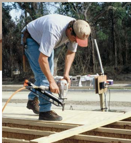
To avoid squeaky floors, use plenty of adhesive and make sure your fasteners don't miss the framing (above). Fully fasten the panels while the adhesive is still wet, using your own weight to provide clamping pressure while you nail (right).
