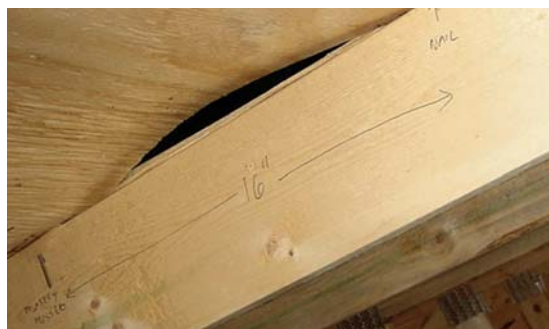
The use of self-spacing H-clips would have prevented this roof sheathing from buckling, which can occur either along the edge (above) or at the end (left) of panels that have been installed without the necessary \frac{1}{8} -inch spacing.
