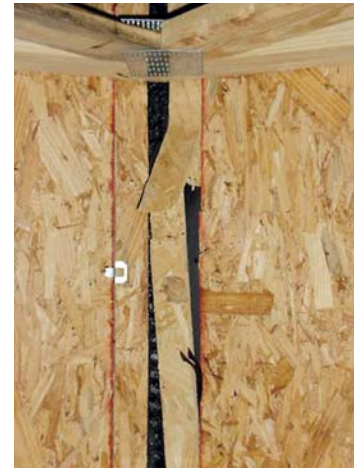
Roof sheathing that's narrower than 24 inches or that doesn't span at least three rafters can feel soft or even break under the weight of a roofer (above right).
