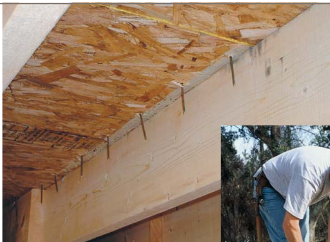
To avoid squeaky floors, use plenty of adhesive and make sure your fasteners don't miss the framing (above). Fully fasten the panels while the adhesive is still wet, using your own weight to provide clamping pressure while you nail (right).
