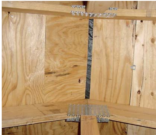
Roof sheathing that's narrower than 24 inches or that doesn't span at least three rafters can feel soft or even break under the weight of a roofer (above right).
