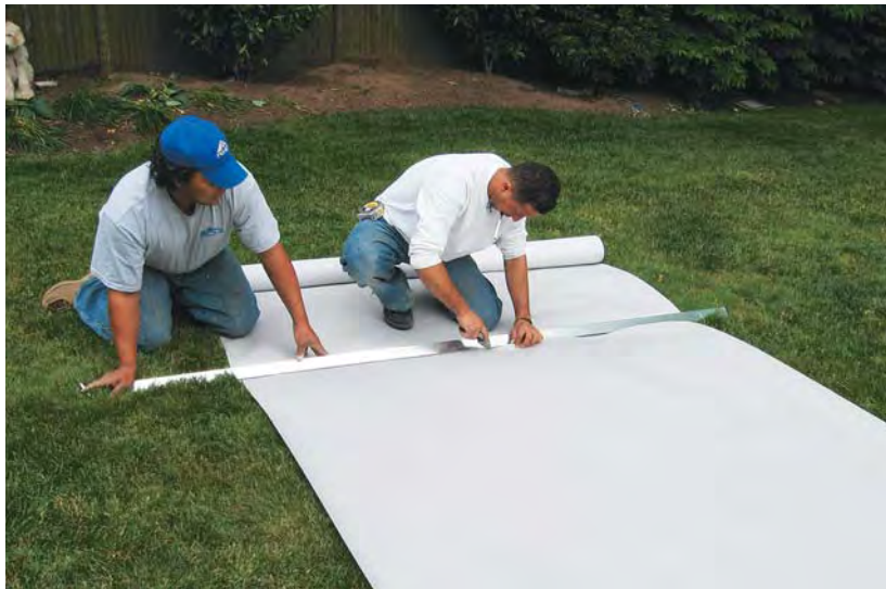
Figure 3. After cutting the first section of membrane to length (right), the installation crew dry-fits it to the deck. Once it's in position, they roll back half the membrane lengthwise (below) and apply adhesive to the exposed part of the deck before laying the membrane back in place (below right).
