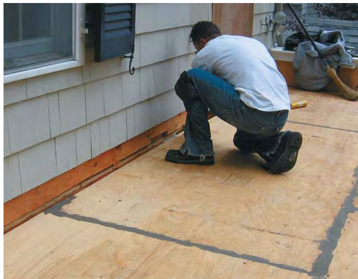
Figure 2. After installing the metal perimeter drip edge, the Duradek installers patch joints, nail heads, and voids in the plywood deck with a silica-based floor filler (above), then sand the deck smooth (above right). Sealant fills the joint between the deck and wall sheathing, preventing the membrane from forming a water-collecting crease (right).
