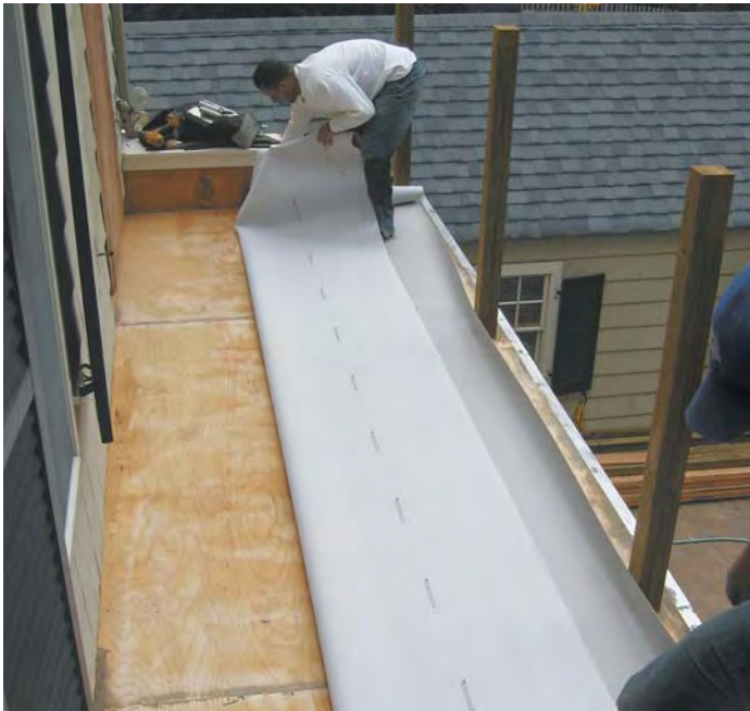
Figure 3. After cutting the first section of membrane to length (right), the installation crew dry-fits it to the deck. Once it's in position, they roll back half the membrane lengthwise (below) and apply adhesive to the exposed part of the deck before laying the membrane back in place (below right).
