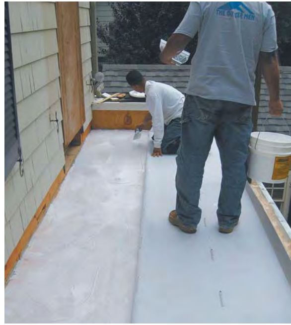
Figure 4. A crew member carefully marks and cuts openings for the rail posts (far left). Then, after gluing down the strip of membrane along the edge of the deck, he glues down the main section of membrane, overlapping the perimeter strip 1 inch (left).
