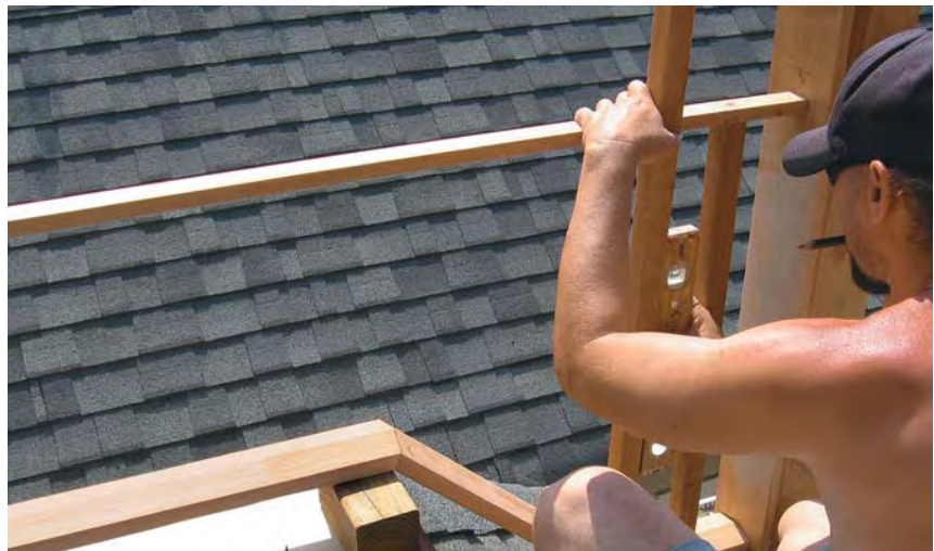
Figure 7. A simple painted cedar railing finishes the deck (left). Balusters are attached with screws through a rail insert at the top (below). A V-shaped notch at the base of each baluster (bottom) matches the beveled top of the shoe rail.
