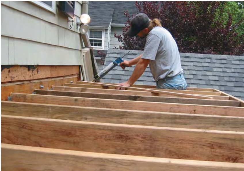
Figure 1. Tapered strips of framing lumber glued and screwed to the deck joists supply the necessary 2 percent slope for drainage (top). Four-by-four PT railing posts are bolted to the framing (right) before the plywood deck sheathing is installed (far right).
