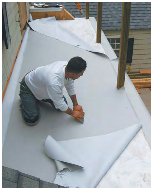
Figure 4. A crew member carefully marks and cuts openings for the rail posts (far left). Then, after gluing down the strip of membrane along the edge of the deck, he glues down the main section of membrane, overlapping the perimeter strip 1 inch (left).
