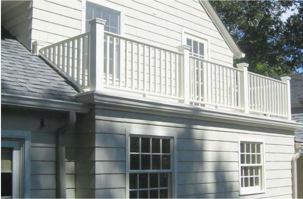
Figure 7. A simple painted cedar railing finishes the deck (left). Balusters are attached with screws through a rail insert at the top (below). A V-shaped notch at the base of each baluster (bottom) matches the beveled top of the shoe rail.
