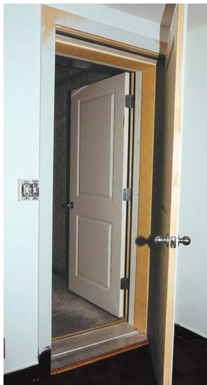
Figure 4. A pair of 1 3 / 4 -inch solid-core doors — air-sealed as carefully as exterior doors — create a sound-defeating air lock between the practice room and the rest of the basement.
