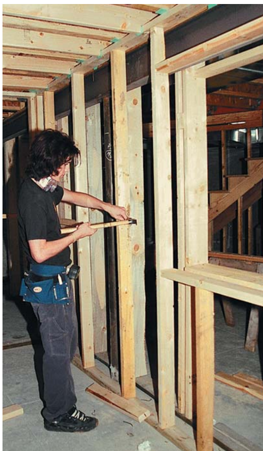
Figure 1. Parallel 2x4 partition walls (left) provide acoustic separation between rooms. To reduce sound transmission to the living space above, the author dropped separate 2x10 ceiling joists below the plane of the I-joist floor system. Note the green PVC gaskets separating the joists from the plates. Before drywall, the crew sealed potential airborne sound paths with caulk and spray foam (below left), then filled the cavities with mineral-wool insulation to further dampen air vibration (below).
