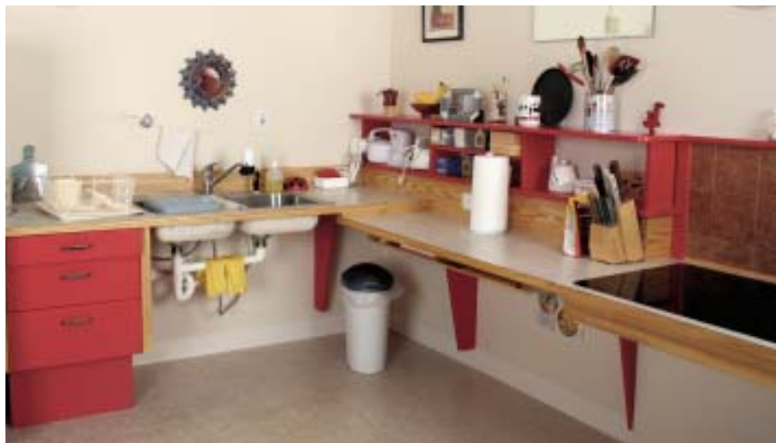
Figure 6. Conveniently located between the sink and the cooktop, the food-prep area features continuous knee space and ample storage in the “margin,” the area just above the countertop.
