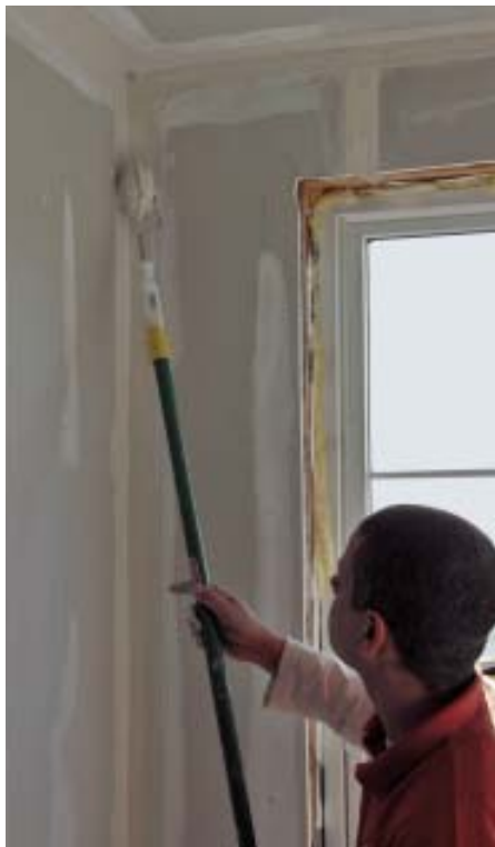
Figure 4. To rapidly finish inside corners, the author submerges a 3-inch lamb's wool paint roller in the bucket of mud (above left), then places the roller in a corner (above right) and applies just enough pressure to evenly coat both sides of the corner at the same time (far right, top). Then he grabs a precut length of tape and presses it into place with his fingers (far right, bottom).
