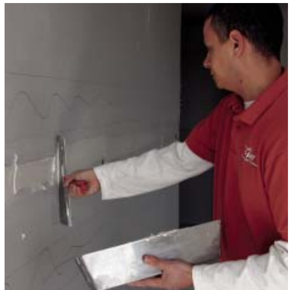
Figure 3. Instead of using a puny tapping knife, the author fully loads a 12-inch broad knife with mud, holds the knife edge parallel to the seam, and covers the tape in one long, sweeping motion (left). To wipe the joint smooth, he holds the knife at a shallow angle and applies gentle but equal pressure to both ends of it (right).
