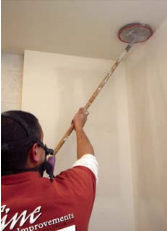
Figure 6. A Radius 360 pole sander covers more ground faster than a standard rectangular sander, and its soft orange bumper won't wear a groove in the corner (left). An angled sponge sander makes quick work of the spot in the corner where the round sander can't reach (above).
