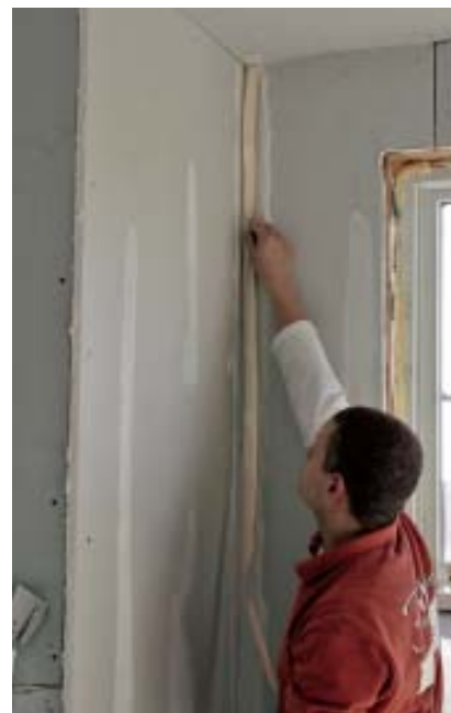
Figure 4. To rapidly finish inside corners, the author submerges a 3-inch lamb's wool paint roller in the bucket of mud (above left), then places the roller in a corner (above right) and applies just enough pressure to evenly coat both sides of the corner at the same time (far right, top). Then he grabs a precut length of tape and presses it into place with his fingers (far right, bottom).
