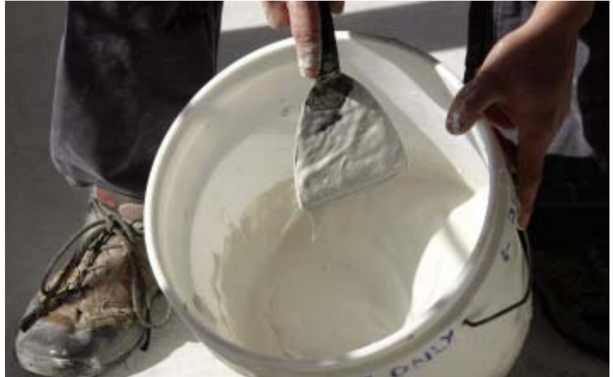
Figure 2. Properly mixed setting-type compound is smooth and lump-free, with the consistency of thick pancake batter.
