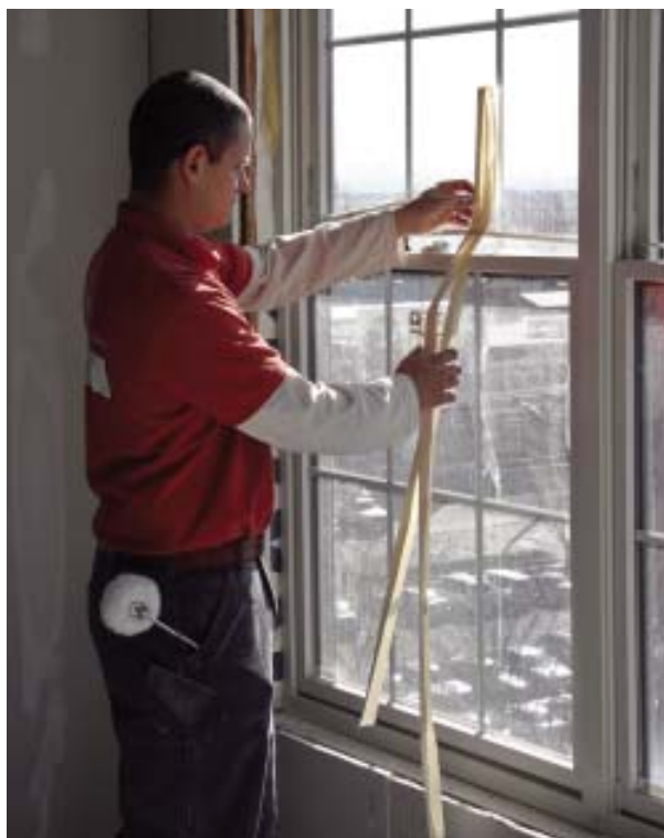
Figure 1. Before mixing joint compound, the author covers all factory-tapered seams with self-adhesive mesh tape (above). For corners, he uses paper tape, which he precuts and precreases to keep the taping process moving quickly (right).
