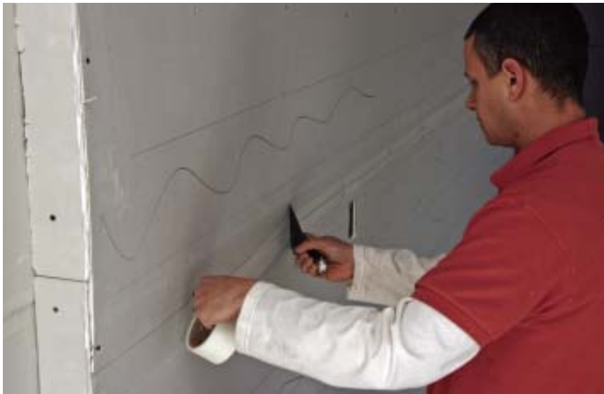
Figure 1. Before mixing joint compound, the author covers all factory-tapered seams with self-adhesive mesh tape (above). For corners, he uses paper tape, which he precuts and precreases to keep the taping process moving quickly (right).
