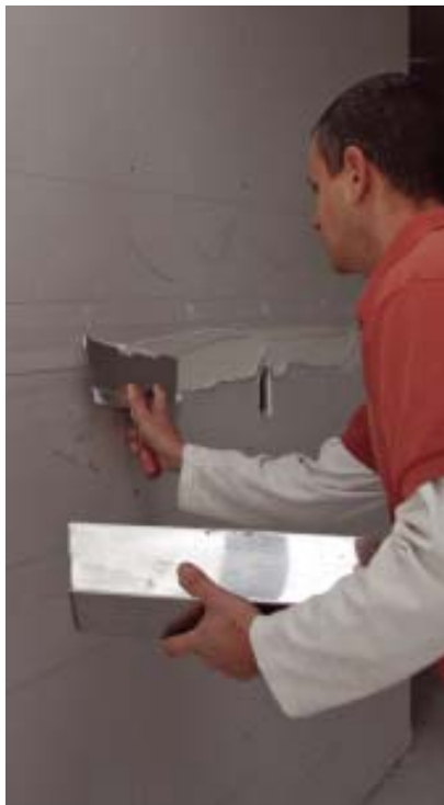
Figure 3. Instead of using a puny tapping knife, the author fully loads a 12-inch broad knife with mud, holds the knife edge parallel to the seam, and covers the tape in one long, sweeping motion (left). To wipe the joint smooth, he holds the knife at a shallow angle and applies gentle but equal pressure to both ends of it (right).
