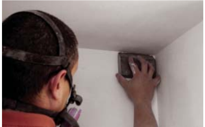
Figure 6. A Radius 360 pole sander covers more ground faster than a standard rectangular sander, and its soft orange bumper won't wear a groove in the corner (left). An angled sponge sander makes quick work of the spot in the corner where the round sander can't reach (above).
