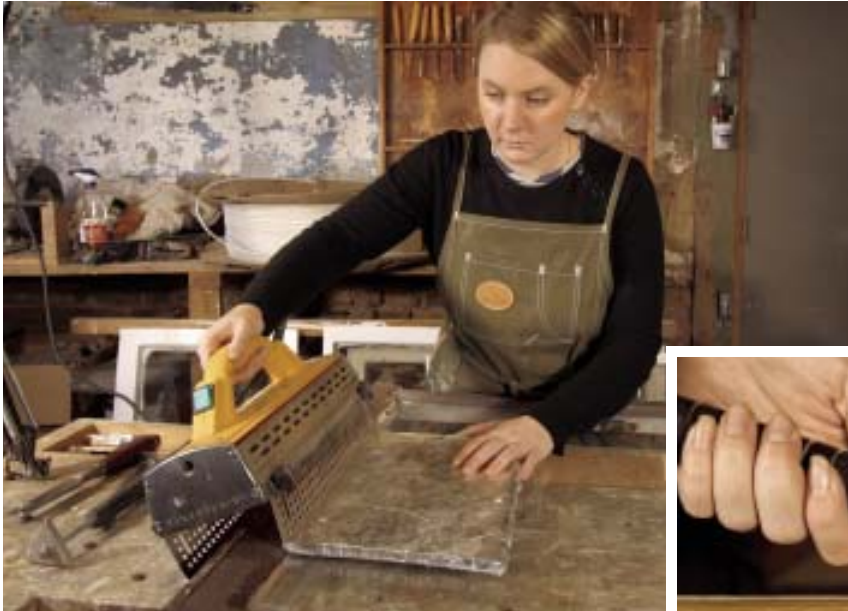
Figure 2. Placed over a heat shield to protect the glass, an infrared paint remover softens up the glazing compound and paint (left). After a minute or so, both materials release their grip on the wood and can be quickly scraped off (below). A special chisel with an adjustable guide wheel removes glazing compound without harming the glass (bottom).
