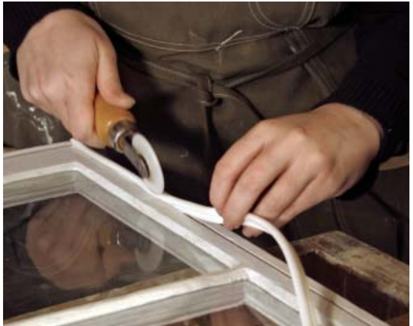
Figure 4. The author prepares a sash to receive weather stripping by routing a 3mm groove into the mating surfaces of the sashes (top). After the sash is fully primed, horizontal surfaces — such as the meeting rail shown above — are fitted with silicone bead. On the exterior of each sash, vertical surfaces are fitted with brush-type weather seals, which seal tightly to the stops but don't interfere with opening and closing.
