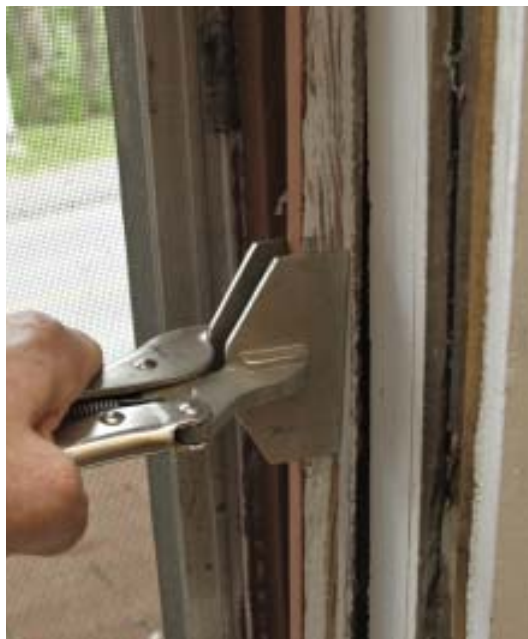
Figure 1. A set of wide-mouth Vise-Grips helps extract parting bead without undue damage.
