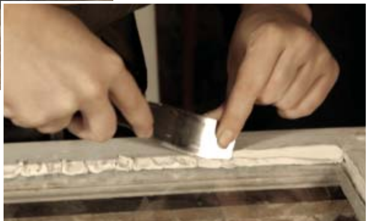
Figure 3. Holding a ball of glazing putty in one hand, a worker tears off manageable chunks and presses them in place with her fingers (above). When one side of the sash is fully loaded, she tools the compound smooth with a glazier's curved putty knife (right).
