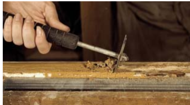
Figure 2. Placed over a heat shield to protect the glass, an infrared paint remover softens up the glazing compound and paint (left). After a minute or so, both materials release their grip on the wood and can be quickly scraped off (below). A special chisel with an adjustable guide wheel removes glazing compound without harming the glass (bottom).
