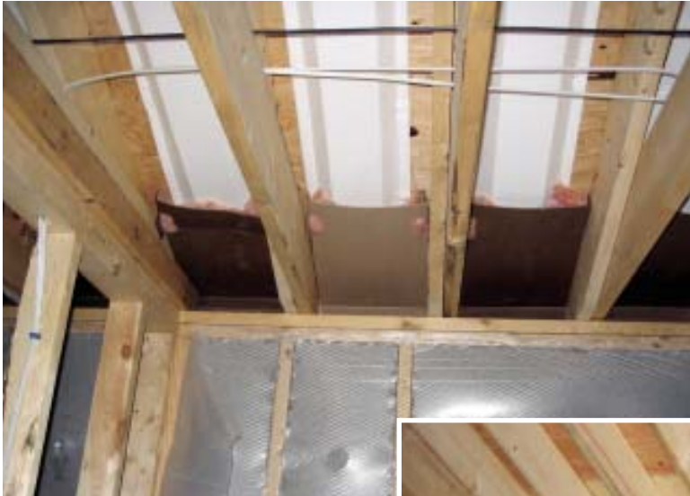
Figure 7. In an effort to prevent windwashing of attic insulation, the author first tried using cardboard baffles above the top plates, then stuffed the gaps between the baffles and the polystyrene ventilation chute with fiberglass batts (left). His discovery of a plastic baffle called AccuVent (below) made this process much easier.
