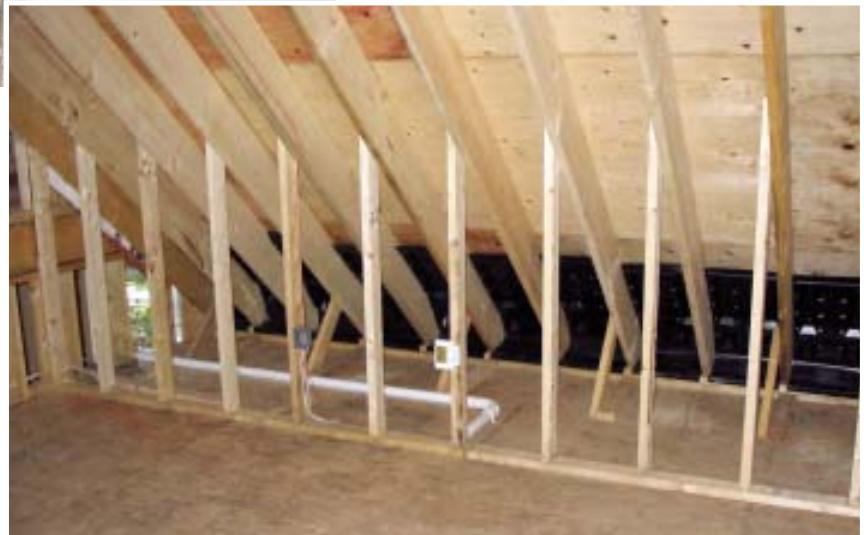
Figure 7. In an effort to prevent windwashing of attic insulation, the author first tried using cardboard baffles above the top plates, then stuffed the gaps between the baffles and the polystyrene ventilation chute with fiberglass batts (left). His discovery of a plastic baffle called AccuVent (below) made this process much easier.
