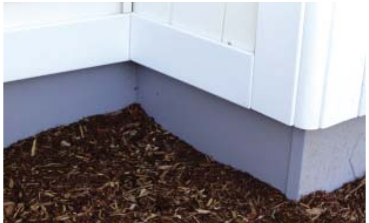
Figure 4. The siding contractor covered the exposed portion of the insulation board with vinyl coil stock. He waited until the job was nearly complete so that the vinyl wouldn’t get damaged by the work in progress.
