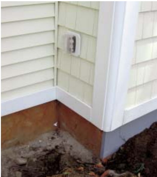
Figure 4. The siding contractor covered the exposed portion of the insulation board with vinyl coil stock. He waited until the job was nearly complete so that the vinyl wouldn’t get damaged by the work in progress.
