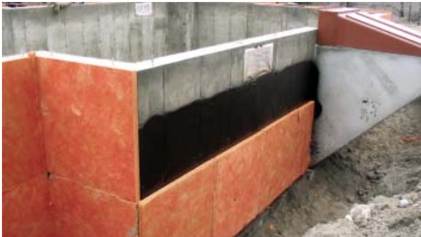
Figure 2. Warm-N-Dri foundation insulation board is pressed into a proprietary spray coating, which holds it in place for backfilling. The fiberglass board acts as a drainage mat and is said to discourage insects.
