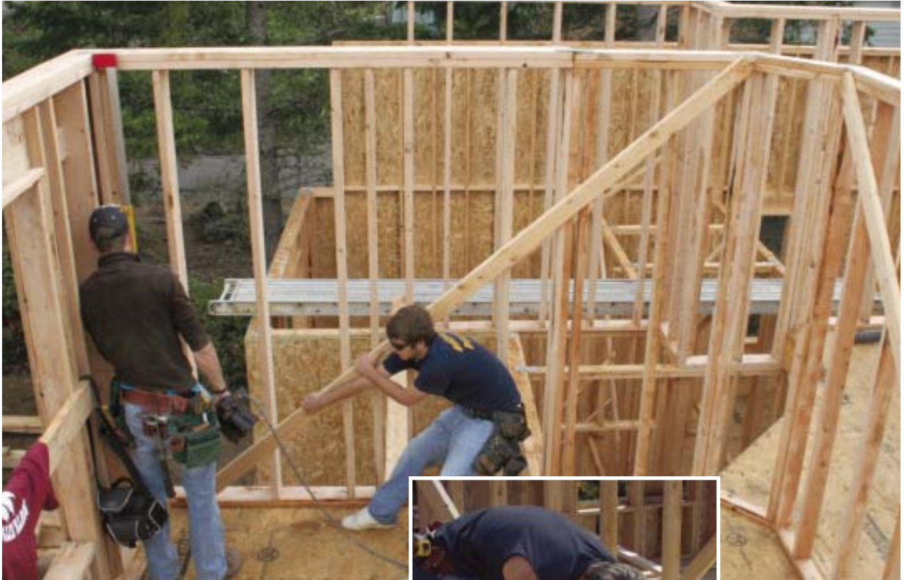
Figure 5. An unsheathed wall can usually be racked square with muscle power alone (above). If the plate doesn't have to go far, it can be pushed into position with a brace nailed on edge (left).
