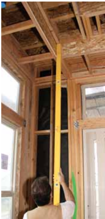
Figure 9. Soffits must be plumb (above) and level (above right). Low joist hangers (right) also have to be fixed.
