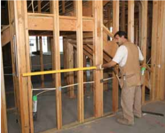
Figure 6. Although parts of this wall (above) have already been planed, the author checks it again for flatness because it will receive wainscot paneling. The junction between floors is a common problem area in stairwells (right); the overhanging subfloor (far right) will have to be trimmed to prevent an obvious bump in the drywall.
