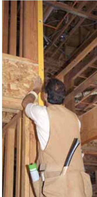
Figure 6. Although parts of this wall (above) have already been planed, the author checks it again for flatness because it will receive wainscot paneling. The junction between floors is a common problem area in stairwells (right); the overhanging subfloor (far right) will have to be trimmed to prevent an obvious bump in the drywall.
