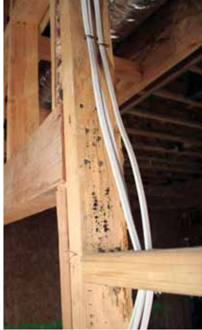
Figure 2. This header (above) and rough sill (above right) will have to be beat or planed flush to the jacks. At right, spray paint indicates doubled studs that need to be planed flush to one another.
