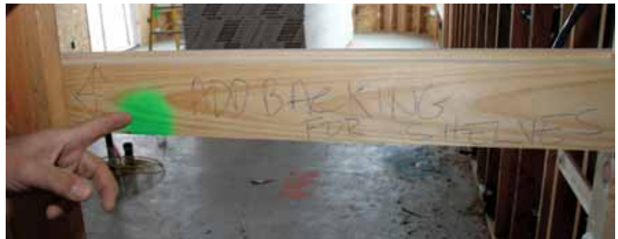
Figure 7. In the bathroom, the author checks the height of the blocking for the toilet-paper holder (left) and leaves a note for the contractor indicating that blocking is needed for linen-closet shelves (above).
