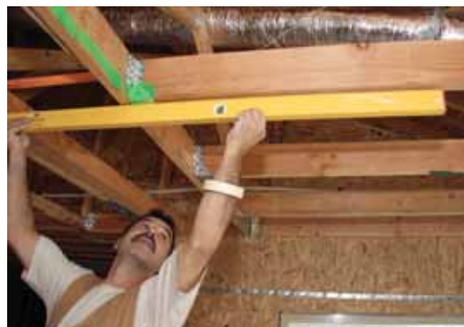
Figure 9. Soffits must be plumb (above) and level (above right). Low joist hangers (right) also have to be fixed.
