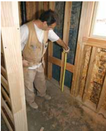
Figure 7. In the bathroom, the author checks the height of the blocking for the toilet-paper holder (left) and leaves a note for the contractor indicating that blocking is needed for linen-closet shelves (above).
