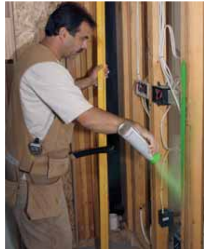
Figure 2. This header (above) and rough sill (above right) will have to be beat or planed flush to the jacks. At right, spray paint indicates doubled studs that need to be planed flush to one another.
