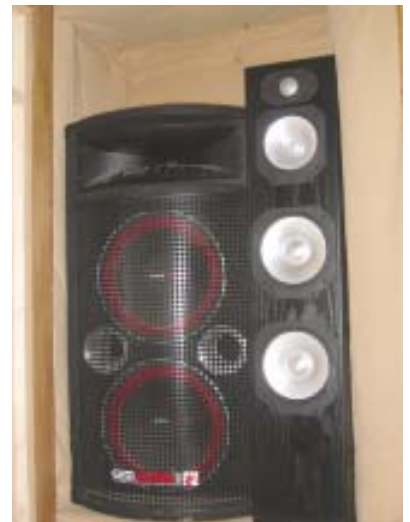
Figure 2. To control low-frequency structure-borne noise, this subwoofer cabinet was lined with a special version of mass-loaded vinyl called NoiseOut 2, which is better at reducing low-frequency noise than conventional loaded vinyl. The material can also be used with hvac equipment and other low-frequency sound sources.
