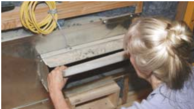
Figure 7. Preventing ducts from spreading sound throughout the house is a two-step process. First, fire-rated acoustic foam or fiberglass duct liner is installed on the ducts' interior to deaden any sound that gets inside (above); next, the ducts' exterior is wrapped (right), which ensures that very little sound will penetrate in the first place. Both steps are especially important in basement home theaters, which often have many ducts in the ceiling.
