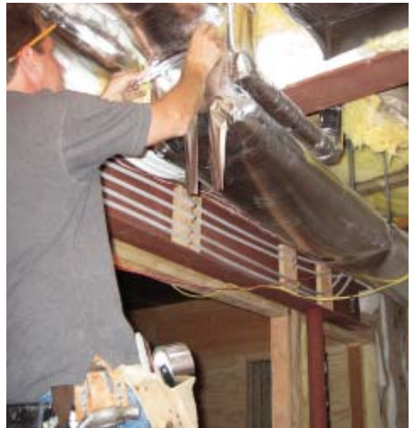
Figure 7. Preventing ducts from spreading sound throughout the house is a two-step process. First, fire-rated acoustic foam or fiberglass duct liner is installed on the ducts' interior to deaden any sound that gets inside (above); next, the ducts' exterior is wrapped (right), which ensures that very little sound will penetrate in the first place. Both steps are especially important in basement home theaters, which often have many ducts in the ceiling.
