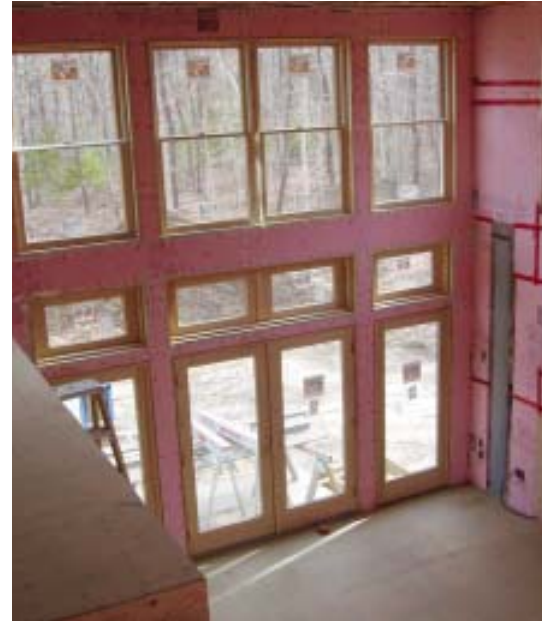
Figure 4. The author blows dense-pack cellulose insulation into wall cavities at about 6 pounds per cubic foot. In 2x6 wall framing, this yields a nominal rating of R-19. Adding a 1-inch layer of polystyrene foam board on the interior, taped at seams, blocks air leakage and vapor transmission and raises the walls to R-24 (above left and above).
