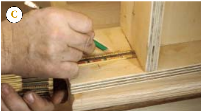
Figure 3. Shopmade handrail stands are the key to the author's assembly system (A) . Screwed to the stairs near the top and bottom, the stands provide support for accurately locating and assembling the hand-railing system in its final position on the finished stair (B) . At the base, the author locates the handrail centerline over the starting baluster center (C, D) , drills through this point, and screws the base to the tread at the first baluster location (E) .
