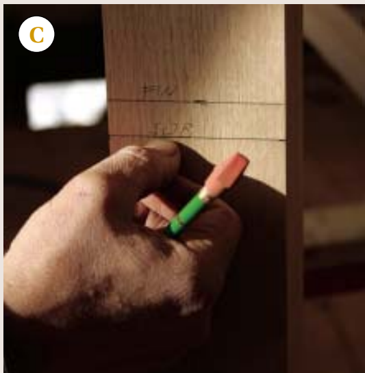
Figure 1. Handrail layout begins with a detailed drawing showing the locations of and relationships between posts, balusters, and treads (A), previous page. The surest way to mark the landing newel for notching is to hold it up in place and refer to full-size drawings made at the planning stage (B). The author marks the finish and subfloor locations on the newel base as the first step in notching the post for installation (C).
