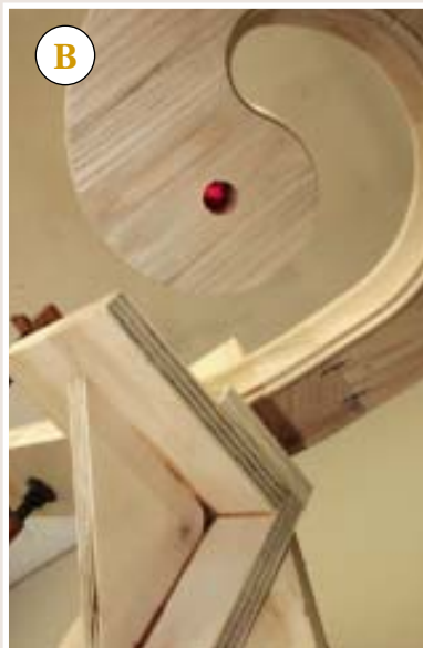
Figure 7. The paper pattern shipped with the volute is fitted to the bullnose tread. The newel center point is targeted with a laser plumb bob (A) and the volute is slid up or down the support platform until its dowel hole is directly centered above the pattern (B). The railing assembly is clamped and marked on the platform for future reference (C). The author punches the newel center mark through the pattern into the finish tread (D).
