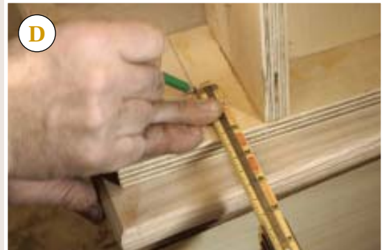
Figure 3. Shopmade handrail stands are the key to the author's assembly system (A) . Screwed to the stairs near the top and bottom, the stands provide support for accurately locating and assembling the hand-railing system in its final position on the finished stair (B) . At the base, the author locates the handrail centerline over the starting baluster center (C, D) , drills through this point, and screws the base to the tread at the first baluster location (E) .
