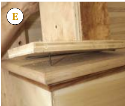
Figure 3. Shopmade handrail stands are the key to the author's assembly system (A) . Screwed to the stairs near the top and bottom, the stands provide support for accurately locating and assembling the hand-railing system in its final position on the finished stair (B) . At the base, the author locates the handrail centerline over the starting baluster center (C, D) , drills through this point, and screws the base to the tread at the first baluster location (E) .
