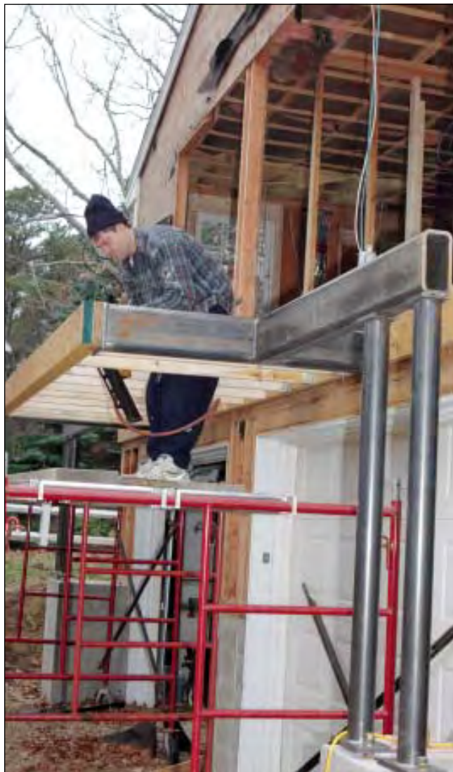
A thick LVL (top), bolted to a welded plate (above), spans the distance between the two post assemblies. Dimensional joists set in hangers (left) run from the LVL to the band at the existing house wall.
