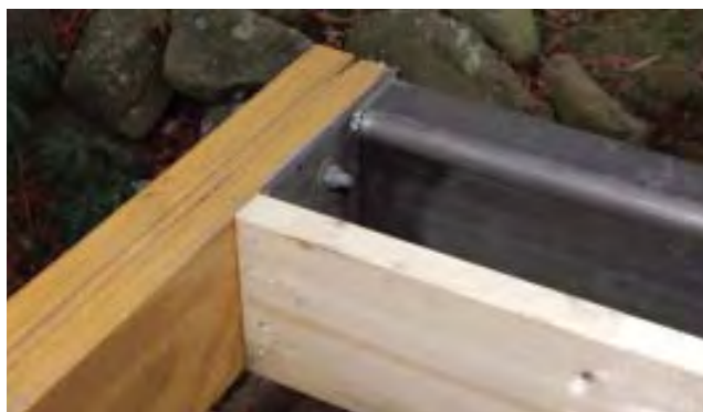
A thick LVL (top), bolted to a welded plate (above), spans the distance between the two post assemblies. Dimensional joists set in hangers (left) run from the LVL to the band at the existing house wall.
