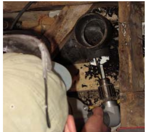
A tradesman prepares to ream the fitting by cutting the existing pipe flush to the face of the hub (above). The end of the Pipe Shredder keeps the bit centered in the pipe. At top right, the bit has been inserted but the cutters have not yet engaged. At right, the cutters have engaged and the bit has gone about ¼ inch into the hub.
