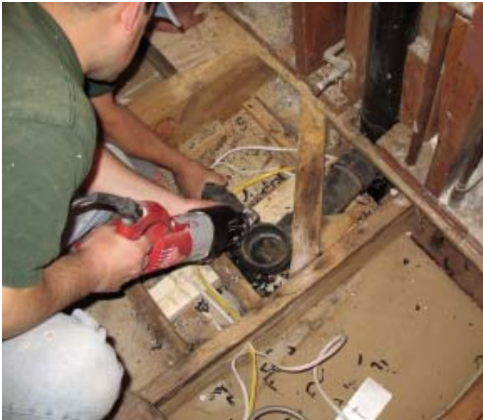
A tradesman prepares to ream the fitting by cutting the existing pipe flush to the face of the hub (above). The end of the Pipe Shredder keeps the bit centered in the pipe. At top right, the bit has been inserted but the cutters have not yet engaged. At right, the cutters have engaged and the bit has gone about ¼ inch into the hub.
