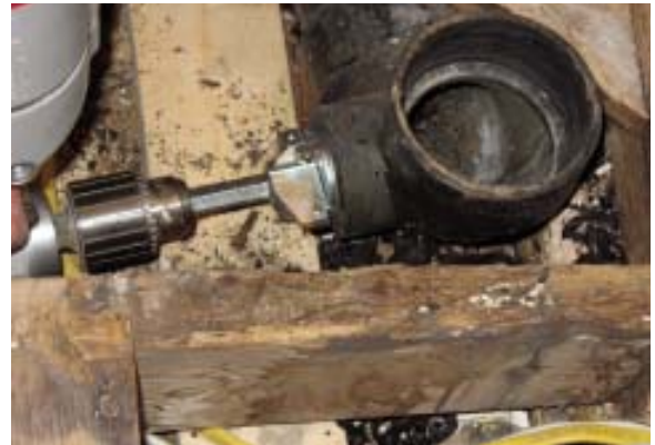
The cutters — which are held in place with screws — cut the pipe as the Pipe Shredder advances into the hub (left). The bits come in a padded case and are sized to fit 1½-, 2-, 3-, and 4-inch pipe (right).
