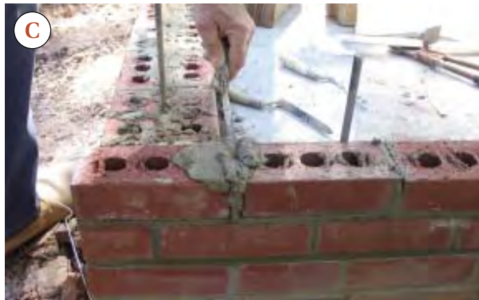
Figure 5. After centering the final “closure” brick in the course (A), the author removes the string line and throws mud down the unmortared joint (B), packs it full with a \frac{3}{8} -inch tuck-pointer so that the head joint is completely filled (C), then cleans up the front of the joint (D).
