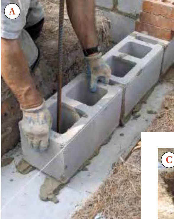
Figure 3. Block courses start at the corners; a string stretched between the two corner blocks helps align the remaining blocks in the course, while pencil marks placed 16 inches on-center on the footing help the author space the blocks properly (A). When setting the last block in the course, he orients it so that the flanged end is dry, which creates a bigger opening that's easier to fill with mortar (B). After setting the block, he throws mud in the joint until it's full (C), then uses a \frac{3}{4} -inch tuck-pointer to pack the joint (D).
