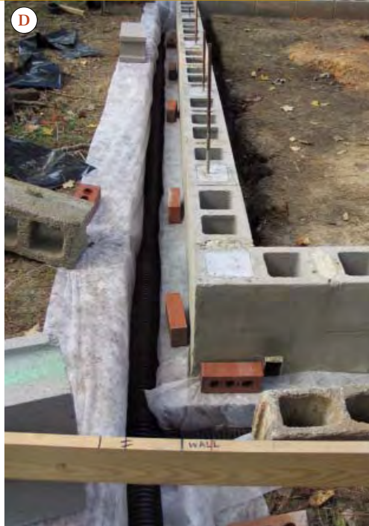
Figure 1. Batter boards and string guide the footing layout. Here, top of slab determines top of footing (A), positioned to allow for two courses of block and two courses of brick. Strings set at the exact center of the wall guide the placement of vertical rebar, every 40 inches, in the wet footing (B). After the footing sets, new strings placed along the outside edge of the wall guide the location of the corners, which the author transfers with a laser (C). Careful layout pays off when the block is laid and the reinforcing is centered in the cores (D).
