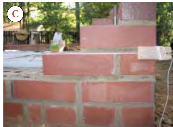
Figure 4. The author uses the edge of his trowel to quickly align the brick that he's laying with the one below (A), then uses a level to make sure the corner is plumb (B). When the mortar has had time to set up, he uses line strings to hold strings (C). Because string tension can pop a freshly laid brick right out of the mortar, he sometimes runs the strings long and uses line twigs as guides (D).
