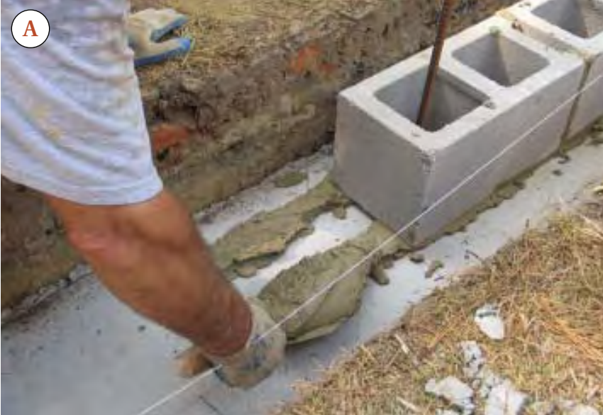
Figure 2. To efficiently spread bed-joint mortar, the author brings his loaded trowel to the footing, gives the trowel a little downward motion, then stops abruptly (A). Next he quickly rotates his wrist while pulling the trowel back, leaving a uniform line of mortar (B). When buttering bricks or blocks, he picks up about half a trowelful of mortar (C), then gives it a good hard shake by thrusting it down and pulling it back up sharply. This flattens the mortar against the trowel (D) so that it will stay put when the trowel is turned over (E).
