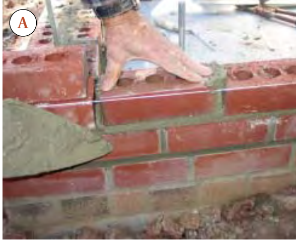
Figure 5. After centering the final “closure” brick in the course (A), the author removes the string line and throws mud down the unmortared joint (B), packs it full with a \frac{3}{8} -inch tuck-pointer so that the head joint is completely filled (C), then cleans up the front of the joint (D).
