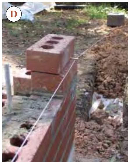
Figure 4. The author uses the edge of his trowel to quickly align the brick that he's laying with the one below (A), then uses a level to make sure the corner is plumb (B). When the mortar has had time to set up, he uses line strings to hold strings (C). Because string tension can pop a freshly laid brick right out of the mortar, he sometimes runs the strings long and uses line twigs as guides (D).
