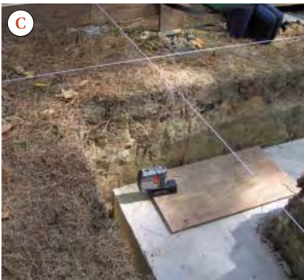
Figure 1. Batter boards and string guide the footing layout. Here, top of slab determines top of footing (A), positioned to allow for two courses of block and two courses of brick. Strings set at the exact center of the wall guide the placement of vertical rebar, every 40 inches, in the wet footing (B). After the footing sets, new strings placed along the outside edge of the wall guide the location of the corners, which the author transfers with a laser (C). Careful layout pays off when the block is laid and the reinforcing is centered in the cores (D).
