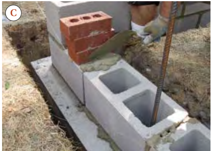
Figure 3. Block courses start at the corners; a string stretched between the two corner blocks helps align the remaining blocks in the course, while pencil marks placed 16 inches on-center on the footing help the author space the blocks properly (A). When setting the last block in the course, he orients it so that the flanged end is dry, which creates a bigger opening that's easier to fill with mortar (B). After setting the block, he throws mud in the joint until it's full (C), then uses a \frac{3}{4} -inch tuck-pointer to pack the joint (D).
