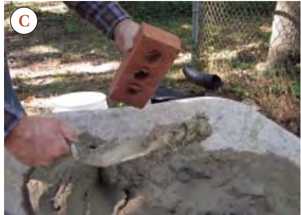
Figure 2. To efficiently spread bed-joint mortar, the author brings his loaded trowel to the footing, gives the trowel a little downward motion, then stops abruptly (A). Next he quickly rotates his wrist while pulling the trowel back, leaving a uniform line of mortar (B). When buttering bricks or blocks, he picks up about half a trowelful of mortar (C), then gives it a good hard shake by thrusting it down and pulling it back up sharply. This flattens the mortar against the trowel (D) so that it will stay put when the trowel is turned over (E).
