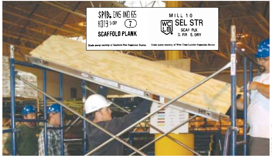
Figure 7. A grade stamp is the only indication that a solid lumber plank is suitable for scaffold use. Readily recognizable engineered scaffold planks, like the aluminum and plywood version shown here, remove any element of doubt.
