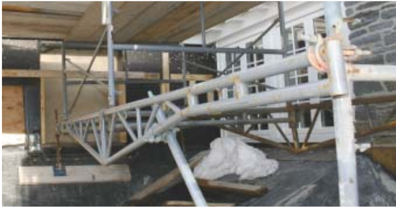
Figure 13. Putlogs — essentially tubular steel trusses — allow you to scaffold around structural obstacles like this projecting roofline (left), or to maintain clear passage beneath a work platform (below). Special brackets connect the putlogs to the frame (below left).
