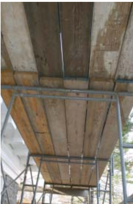
Figure 14. Full planking prevents sideways shifts and treacherous gaps in the platform.
