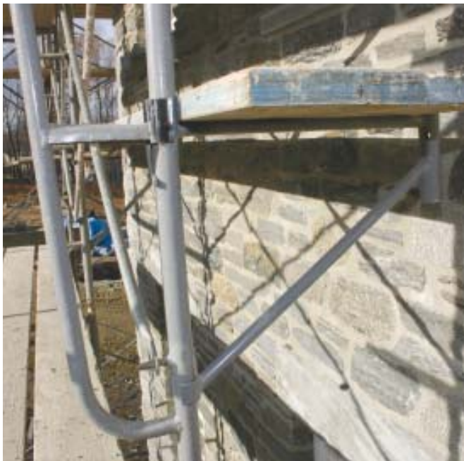
Figure 10. Side arms (above) extend the width of the platform and may be offset from the main platform for working convenience. Frame ledgers provide height adjustment in 16-inch increments.
