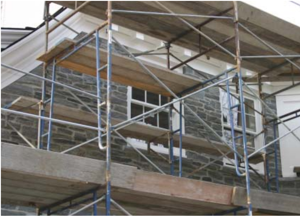
Figure 3. Pipe frames come in several configurations for staging various building heights. Here, short ledger frames are stacked above taller, walk-through frames on a multilevel scaffold.
