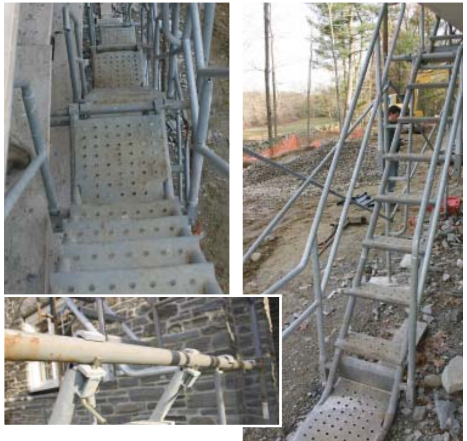
Figure 4. Stair systems provide safe scaffold access when ladders are impractical. Handrails install separately and should never be omitted. Hooks and locking pins secure stair components to the frame (above left). The starting tread of a scaffold stair system or any platform access should be no higher than 24 inches above the base level.
