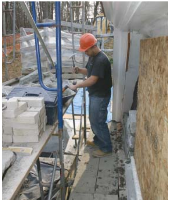
Figure 10. Side arms (above) extend the width of the platform and may be offset from the main platform for working convenience. Frame ledgers provide height adjustment in 16-inch increments.
