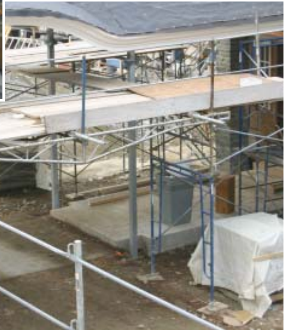
Figure 13. Putlogs — essentially tubular steel trusses — allow you to scaffold around structural obstacles like this projecting roofline (left), or to maintain clear passage beneath a work platform (below). Special brackets connect the putlogs to the frame (below left).
