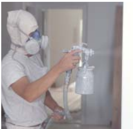
Figure 4. Whether you’re brushing or spraying, the secret to achieving an oil-like finish with a waterborne paint is to apply an even, full coat and keep moving.
