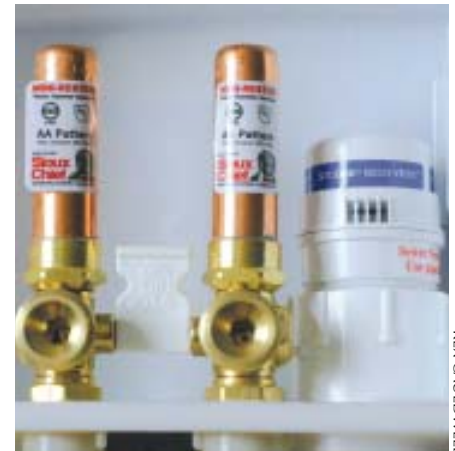
Figure 5. Fitting easily inside a laundry box, a small AAV is a good choice for venting a washing machine. This one connects to a 2-inch trap, which drains into a 3-inch branch line.
