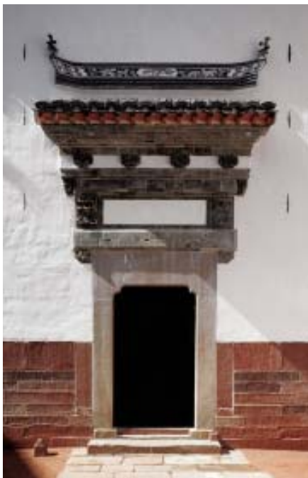
Yin Yu Tang's formal entrance penetrates a stone and brick masonry curtain wall.
