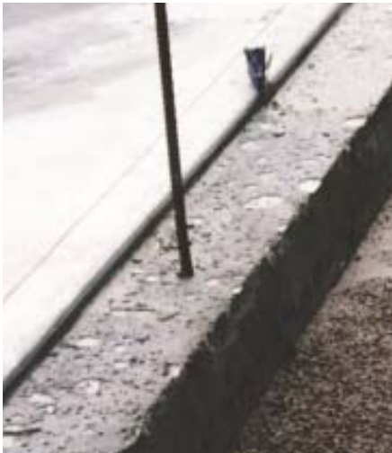
Figure 10. To help block walls store greater amounts of incidental water and to direct the moisture back outside rather than allowing it to trickle into the home, foundations should have a stepped-down shelf at the slab edge. A weep screed at the lower termination of the stucco will allow accumulated water to get out.
