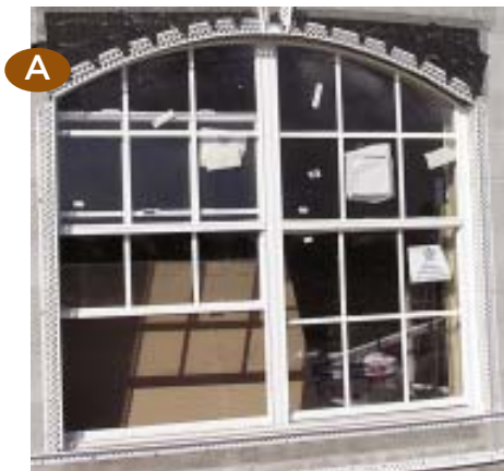
Figure 7. Factory-assembled windows like this double unit (A) are frequently found to leak at the corners (B) and the center joint (C).
