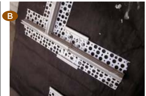
Figure 5. The joint detail typically required in Florida between upper-wall and lower-wall stucco sections (A) does not manage water well. When the control-joint accessory is installed over the top of a continuous sheet of building paper or housewrap (B), water is not kicked to the exterior but is allowed to pass behind the joint into the wall below (C).
