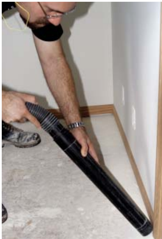
Figure 1. To make sure construction dust won't end up embedded in the finish, the author hits baseboards with a blast of compressed air, followed by thorough vacuuming. The first coat of sanding sealer requires the lion's share of the prep work.
