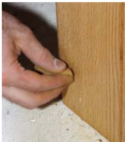
Figure 8. After spraying the sealer coat, the author uses colored putties to fill nail holes. The putty can be intermixed to obtain a close match with the finish work. The author adds whiting to absorb the oil in the putty, thereby preventing wetting of the surrounding wood. Waterborne lacquer doesn't adhere to oil.
