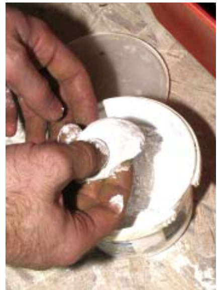
Figure 8. After spraying the sealer coat, the author uses colored putties to fill nail holes. The putty can be intermixed to obtain a close match with the finish work. The author adds whiting to absorb the oil in the putty, thereby preventing wetting of the surrounding wood. Waterborne lacquer doesn't adhere to oil.
