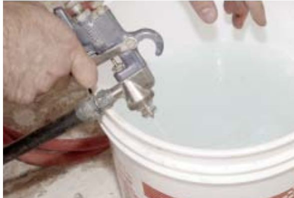
Figure 7. It's important to thoroughly flush the hose and gun between sealer and top coats, as well as on completion of spray operations. Clean water is all that's required, followed by a flush of solvent alcohol to aid drying.
