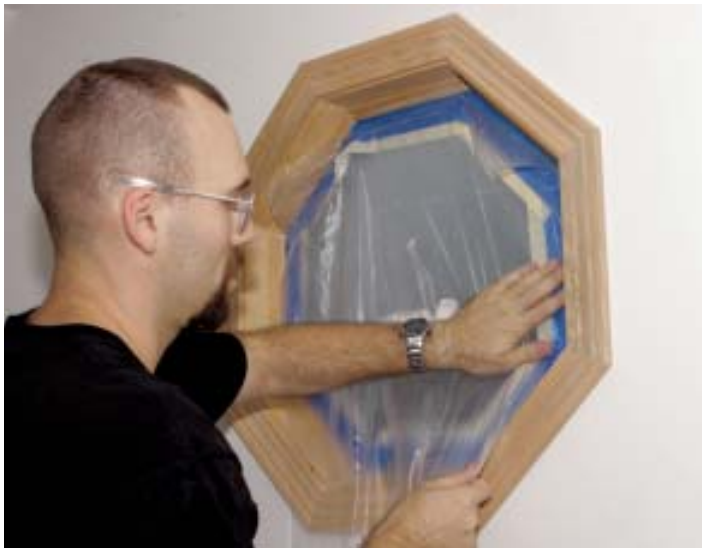
Figure 2. The lacquer goes on the trim before the walls and ceiling are painted, so masking is primarily limited to protecting window glass (above). However, closet ceilings are considered finished after the drywall primer and top coat, so a little extra protection is called for in these areas (right).
