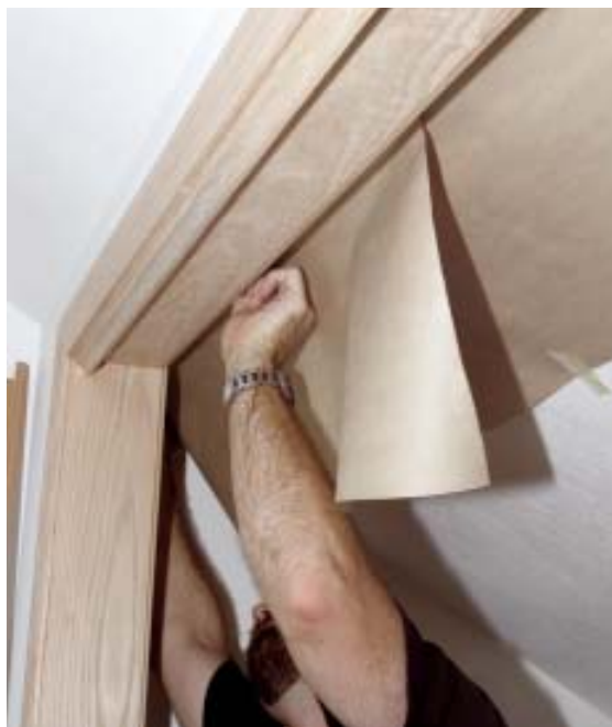
Figure 2. The lacquer goes on the trim before the walls and ceiling are painted, so masking is primarily limited to protecting window glass (above). However, closet ceilings are considered finished after the drywall primer and top coat, so a little extra protection is called for in these areas (right).
