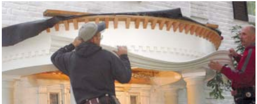
Figure 8. Triangular blocks cut from 2x4s and installed with construction adhesive were pinned to the roof sheathing (left); they provide backing for the flexible crown molding used to finish the portico (below). To place the joints in a less visible position, the author and his helper installed the longest section in the middle, then the two sides (bottom).
