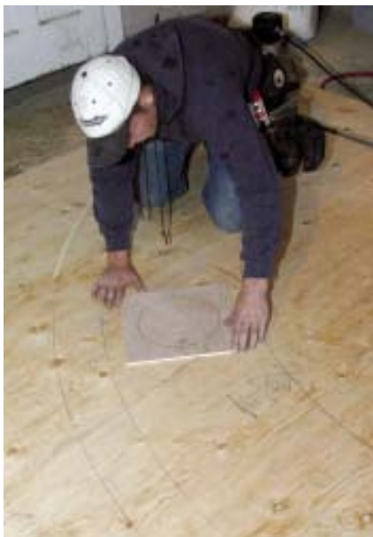
Figure 2. Because the portico's architectural details were drawn to full scale, it was possible to locate columns and plan the framing without using complicated math (left). After cutting out the two sections of the plywood plate with the trammel-mounted router, the author fastened them to the layout table (above) before laying out and precutting the framing.
