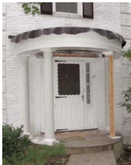
Figure 6. To meet local building-code requirements for wind loads, the author attached brackets (above) to the concrete porch; they will be hidden by the hollow composite columns supporting the portico (right). High-strength aircraft cable running up through the columns connects the brackets to the rafters overhead.
