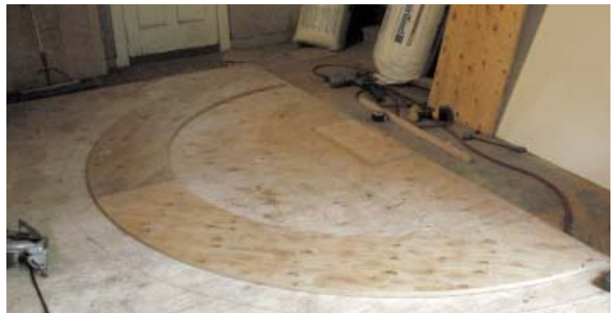
Figure 2. Because the portico's architectural details were drawn to full scale, it was possible to locate columns and plan the framing without using complicated math (left). After cutting out the two sections of the plywood plate with the trammel-mounted router, the author fastened them to the layout table (above) before laying out and precutting the framing.
