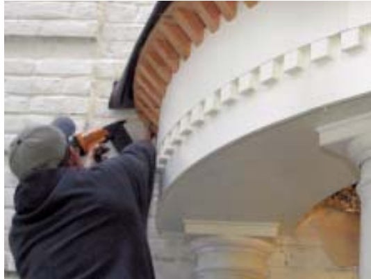
Figure 8. Triangular blocks cut from 2x4s and installed with construction adhesive were pinned to the roof sheathing (left); they provide backing for the flexible crown molding used to finish the portico (below). To place the joints in a less visible position, the author and his helper installed the longest section in the middle, then the two sides (bottom).
