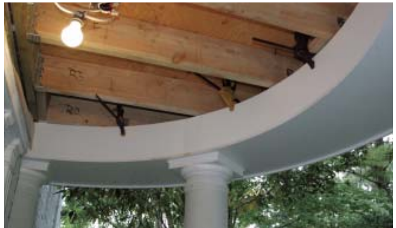
Figure 7. To avoid fracturing the curved interior trim with fasteners, the author coaxed the pieces into position with clamps, allowing friction to hold everything in place (right). He used a base-cap offcut to scribe the beadboard ceiling planks to fit (below left), starting with the longest board in the middle and working toward the two corners (below right).
