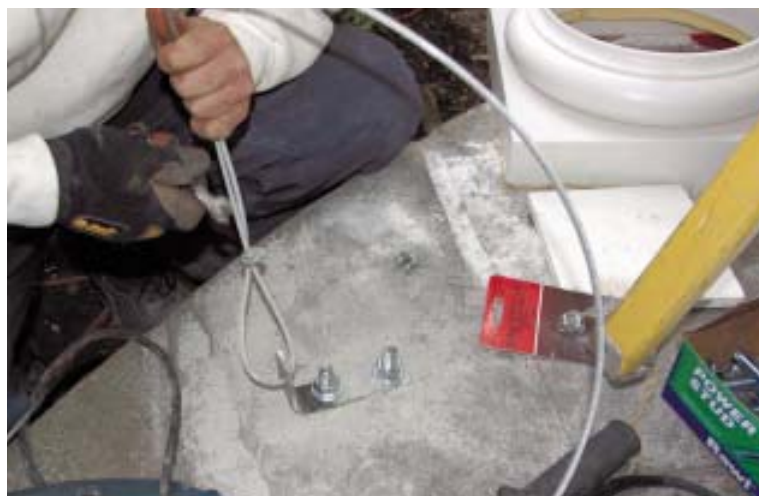
Figure 6. To meet local building-code requirements for wind loads, the author attached brackets (above) to the concrete porch; they will be hidden by the hollow composite columns supporting the portico (right). High-strength aircraft cable running up through the columns connects the brackets to the rafters overhead.
