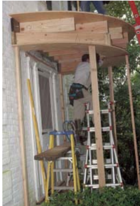
Figure 3. With the plate temporarily supported by 2x4 posts and the precut framing assembled, the roof sheathing was installed as a single piece (above). To provide backing for the two staggered layers of curved plywood sheathing, the author will install 2x4 cripples 6 inches o.c. (not shown) between the bottom plate and the roof sheathing (right).
