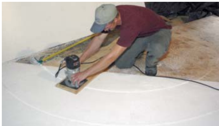
Figure 4. Cut from a 4-foot-by-8-foot sheet of \frac{1}{2} -inch Azek PVC stock, this two-piece matching base cap will be installed under the plywood plate to create a finished soffit.
