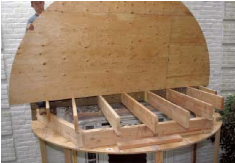
Figure 3. With the plate temporarily supported by 2x4 posts and the precut framing assembled, the roof sheathing was installed as a single piece (above). To provide backing for the two staggered layers of curved plywood sheathing, the author will install 2x4 cripples 6 inches o.c. (not shown) between the bottom plate and the roof sheathing (right).
