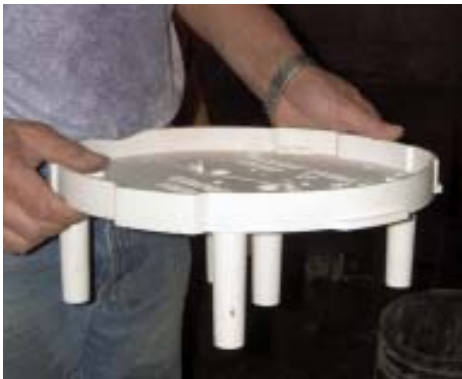
Figure 5. A plastic stand (above) raises the pump about 6 inches above the basket's bottom so it doesn't clog with sediment. Flexible couplings on the discharge line (right) and a two-piece lid (far right) allow the pump to be removed without cutting the pipe.
