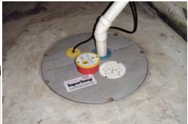
Figure 9. Many customers opt to finish the basement walls with white fiberglass-reinforced panels (left), a big improvement over the moldy masonry typically found in wet basements. The panels are fastened with drive anchors instead of adhesive, leaving space for seeping water to drain to the WaterGuard piping. These pictures were taken only a few days after the sump was installed. Note that the floor is completely dry (above).
