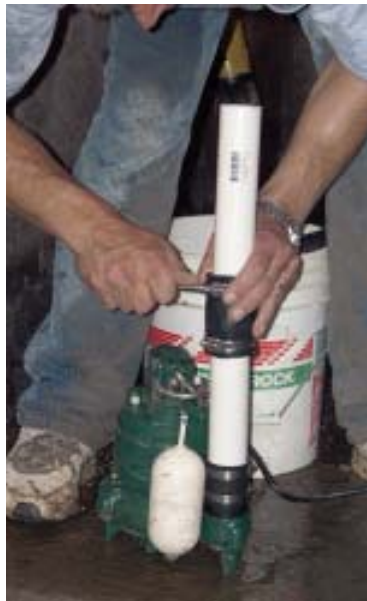
Figure 5. A plastic stand (above) raises the pump about 6 inches above the basket's bottom so it doesn't clog with sediment. Flexible couplings on the discharge line (right) and a two-piece lid (far right) allow the pump to be removed without cutting the pipe.
