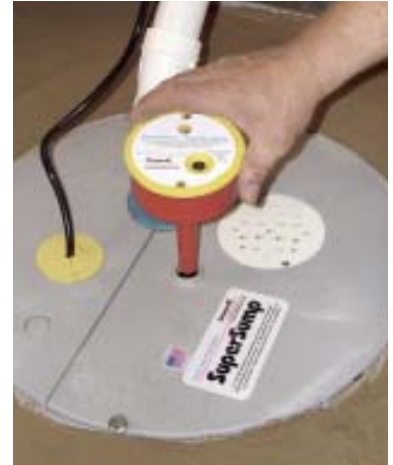
Figure 8. Final steps include patching the floor around the sump and basement perimeter (left) and installing a high-water alarm (above) that sounds when the pump or discharge line malfunctions. An emergency floor drain handles leaks — plumbing mishaps, a broken washing-machine hose, and the like.
