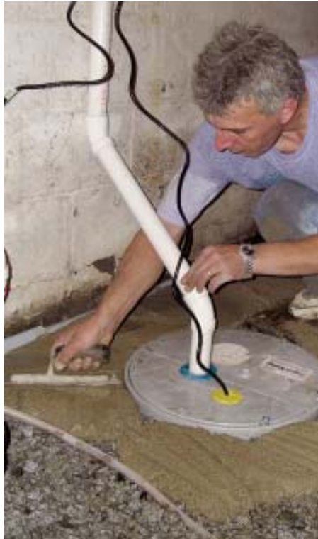
Figure 8. Final steps include patching the floor around the sump and basement perimeter (left) and installing a high-water alarm (above) that sounds when the pump or discharge line malfunctions. An emergency floor drain handles leaks — plumbing mishaps, a broken washing-machine hose, and the like.
