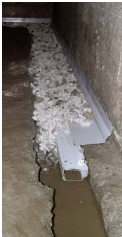
Figure 3. The author uses two styles of proprietary pipe. The standard type (above) is placed against the foundation wall. It has a toothed flange that creates a small gap between the basement wall and slab so any water seeping through the block is directed into the pipe. The job described here required the two-piece version (left) because the footing prevented placing the pipe against the wall. The piping is sloped toward the pump (below) — \frac{1}{4} inch over the length of the wall is usually enough.
