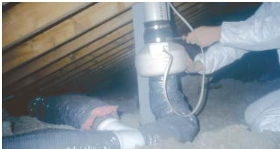
Figure 13. The author often installs a remote-mounted inline fan (above) to provide ventilation for one or more bathrooms, as well as for the whole house. A programmable control is set to provide the correct flow based on the number of occupants and the house's infiltration rate. The author verifies the fan's rated capacity with a flow meter (right).
