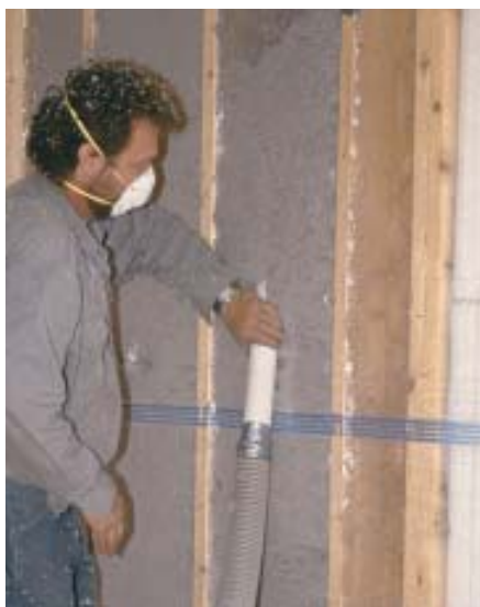
Figure 9. Blowing the wall from the center down, then up, ensures complete filling. A rigid extension wand enables the author to blow to the extremes and gradually withdraw as the cavity fills.
