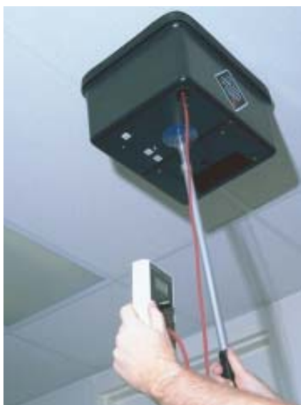
Figure 13. The author often installs a remote-mounted inline fan (above) to provide ventilation for one or more bathrooms, as well as for the whole house. A programmable control is set to provide the correct flow based on the number of occupants and the house's infiltration rate. The author verifies the fan's rated capacity with a flow meter (right).
