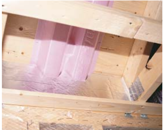
Figure 6. If ceiling bays aren't end-blocked, soffit air can travel below the ceiling insulation and neutralize its function. Piling on more insulation does nothing to correct a cold ceiling complaint (left). Rigid foam blockers, cut to fit around standard insulation baffles, direct ventilation above the ceiling insulation and prevent cold air infiltration (above).
