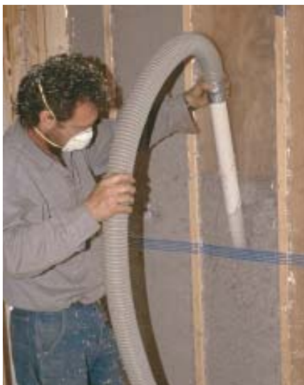
Figure 9. Blowing the wall from the center down, then up, ensures complete filling. A rigid extension wand enables the author to blow to the extremes and gradually withdraw as the cavity fills.
