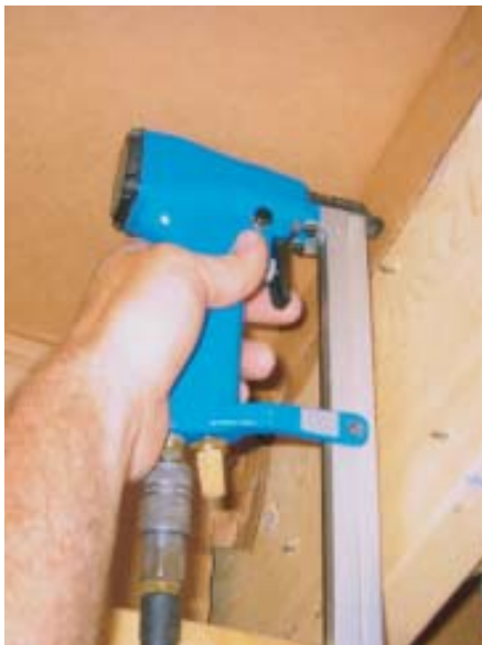
Figure 8. The author uses full-width vapor-permeable cardboard chutes in cathedral ceilings rather than rigid foam baffles. A bend in the bottom piece allows it to act as a wind stop at the top plate.
