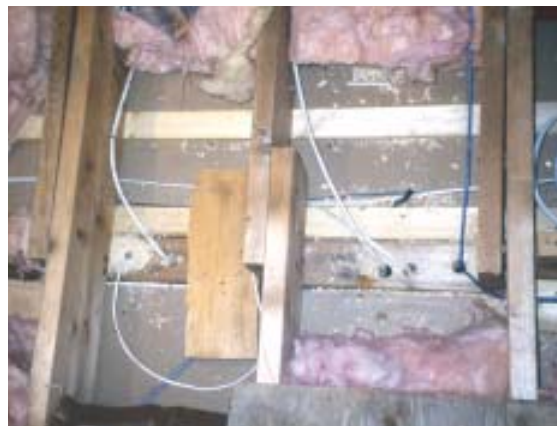
Figure 7. Interior partitions can be leakier than exterior walls, as cold attic air bypasses the top plate through cracks behind drywall and wire or pipe penetrations (drawing, top; photo, left). In remedial work, the author seals the plate with two-part expanding foam to prevent convective looping inside the wall (photo, above).
