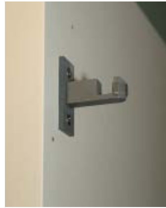
Figure 9. Part of the door interlock is bolted to the inside of the door to the cab. When the elevator is activated, the interlock latches on to the door and won't let go. It releases upon arrival but can be manually opened in an emergency.
