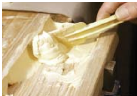
Figure 2. Once the prepared blank has been “battered” with a hard-setting filler, the molding is pressed into place with a vise to form a perfectly detailed negative pattern.
