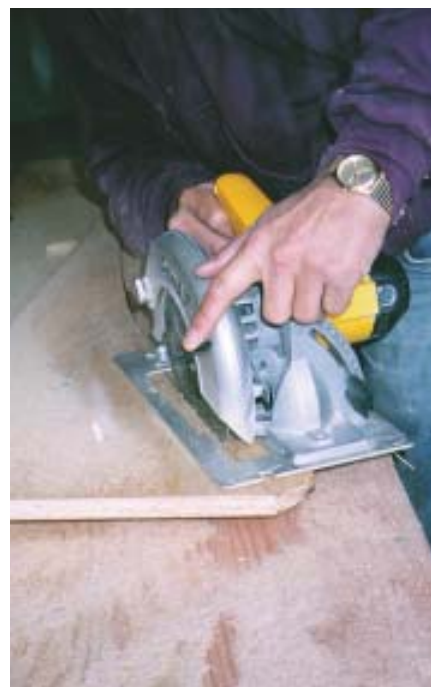
Figure 3. The plywood diagonal arches were cut with a circular saw, which can make faster cuts than a jig saw, down to a 4-foot radius, before binding. Here, a carpenter adds a block to support a center light fixture.
