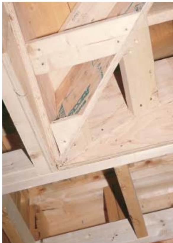
Figure 5. The bevel for the starter block — 26\frac{1}{2} degrees — was the simplest to establish, using a bevel gauge and a miter saw. The rest of the bevels were deduced from that angle.
