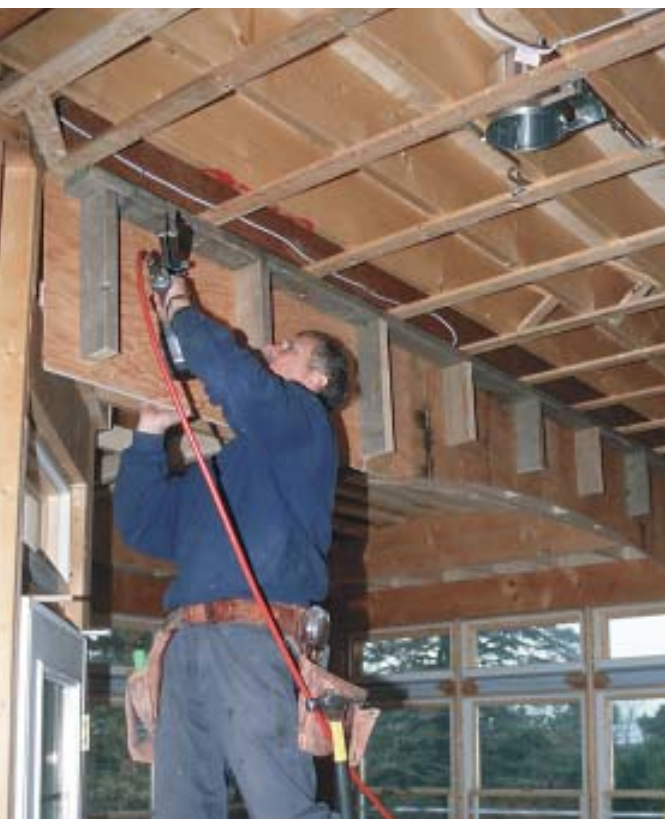
Figure 7. Roughed out on sawhorses and nailed up in two pieces, the box beam's arch had to remain shallow to clear windows at both ends (left). The arch effectively echoes the barrel vault arches and helps to delineate the open but separate living spaces.
