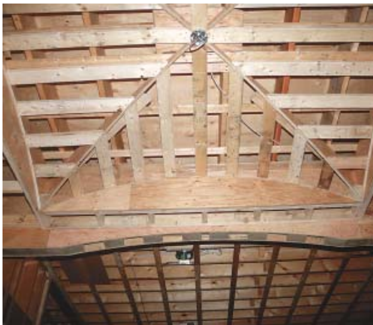
Figure 7. Roughed out on sawhorses and nailed up in two pieces, the box beam's arch had to remain shallow to clear windows at both ends (left). The arch effectively echoes the barrel vault arches and helps to delineate the open but separate living spaces.
