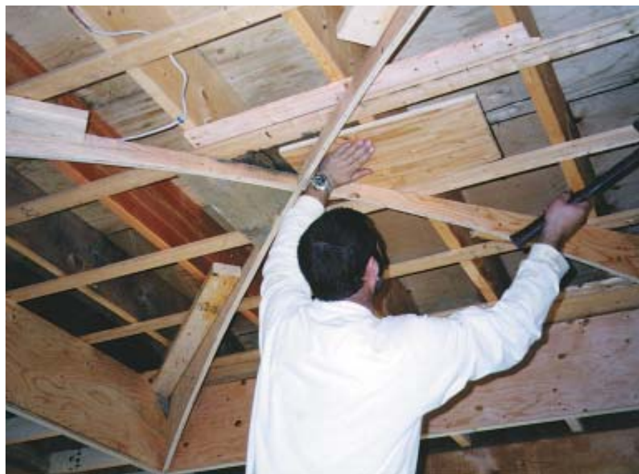
Figure 3. The plywood diagonal arches were cut with a circular saw, which can make faster cuts than a jig saw, down to a 4-foot radius, before binding. Here, a carpenter adds a block to support a center light fixture.
