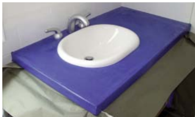
Figure 6. These faucet holes are formed by PVC pipe set into a piece of rigid foam. The foam covers an opening in the plywood and makes that part of the counter thinner so the plumber has plenty of thread to install fixtures.
