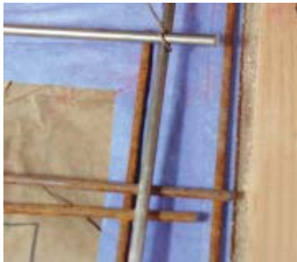
Figure 7. It's important to properly reinforce concrete counters. Here, the form carpenter cuts 6x6 wire mesh around the opening for a drop-in sink. The wire on the back wall will reinforce the integral backsplash. Stainless-steel pencil rod (right) provides extra reinforcement at high-stress areas around the sink opening and along the nosing.
