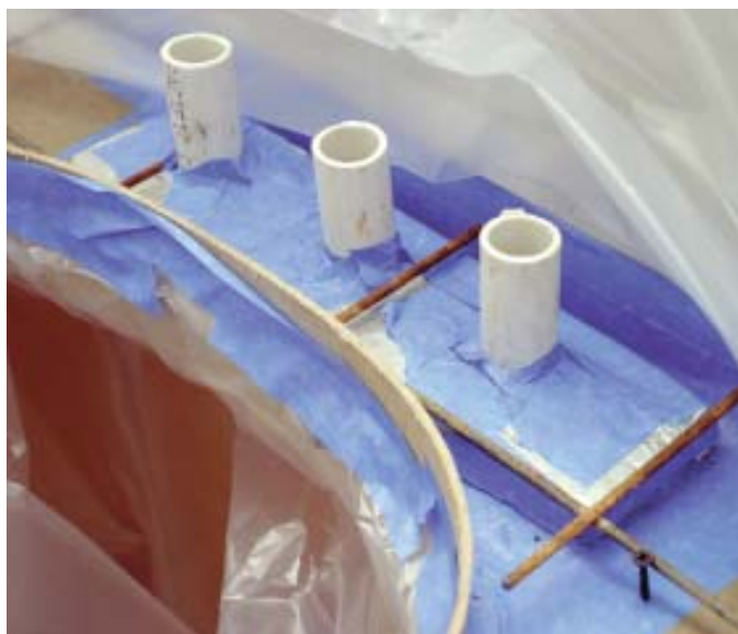
Figure 6. These faucet holes are formed by PVC pipe set into a piece of rigid foam. The foam covers an opening in the plywood and makes that part of the counter thinner so the plumber has plenty of thread to install fixtures.
