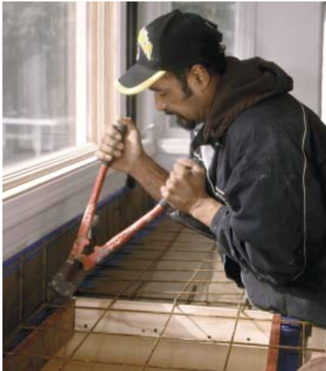
Figure 7. It's important to properly reinforce concrete counters. Here, the form carpenter cuts 6x6 wire mesh around the opening for a drop-in sink. The wire on the back wall will reinforce the integral backsplash. Stainless-steel pencil rod (right) provides extra reinforcement at high-stress areas around the sink opening and along the nosing.
