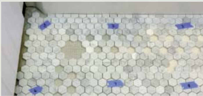
Figure 6. Before spreading any thinset, the author dry-lays the entire floor. This gets all of the tricky cutting done before the wet-setting begins. He labels each mosaic square in sequence so that installation proceeds smoothly. Note the missing accent tiles.
