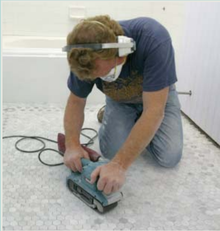
Figure 8. Rather than fuss with leveling the irregular stone tiles from below with extra thinset, the author smooths out any unevenness in the surface with a belt sander.
