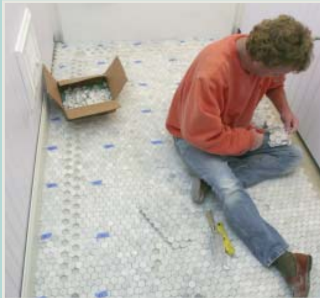
Figure 6. Before spreading any thinset, the author dry-lays the entire floor. This gets all of the tricky cutting done before the wet-setting begins. He labels each mosaic square in sequence so that installation proceeds smoothly. Note the missing accent tiles.
