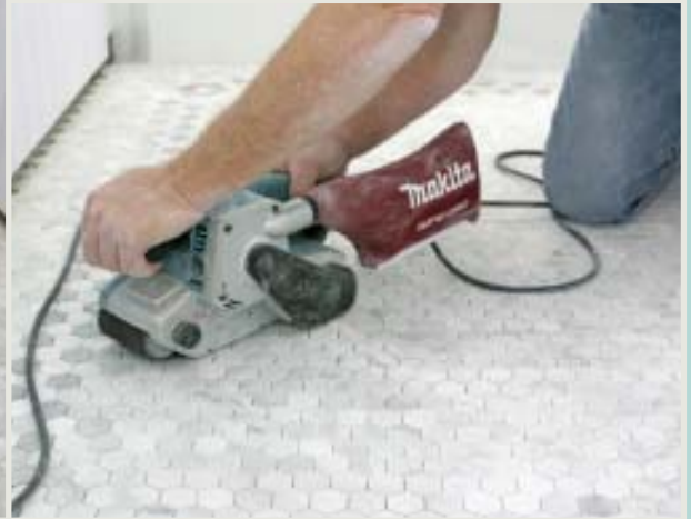
Figure 8. Rather than fuss with leveling the irregular stone tiles from below with extra thinset, the author smooths out any unevenness in the surface with a belt sander.
