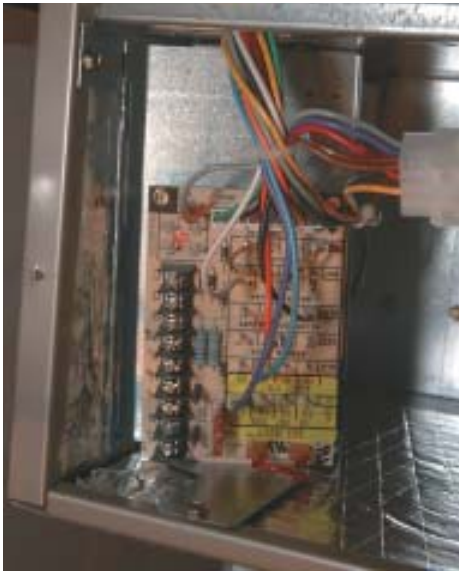
Figure 3. Inside the house, the author installs a variable-speed air handler that is matched to the outdoor condenser. Controlled by advanced electronic circuitry, the air handler's motor can continually adjust to changing loads, ramp up and down gradually as needed, and even sense and adjust to changes in static pressure in the duct system.
