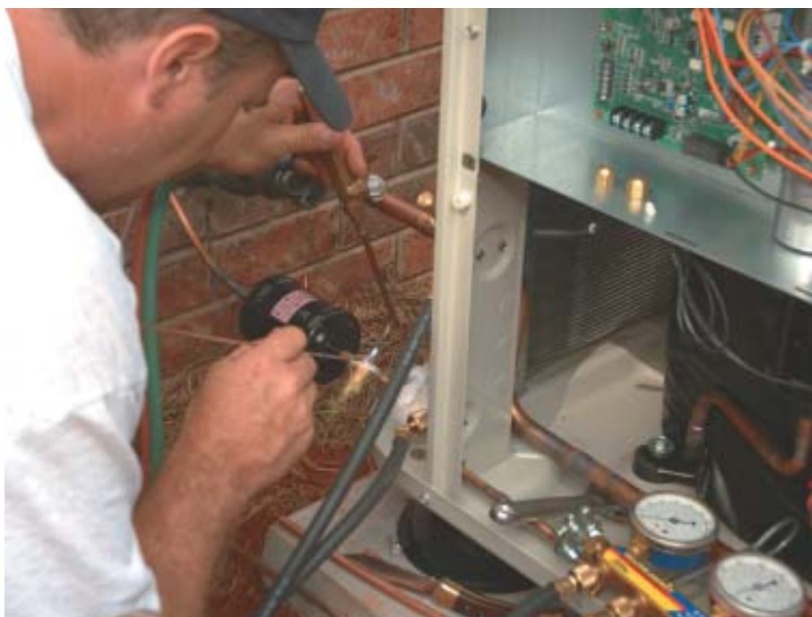
Figure 6. Careful installation work is key to any system's success. Here, the author makes a brazed joint in a copper refrigerant line as he installs a refrigerant dryer that will protect the system against moisture and corrosion.
