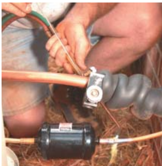
Figure 6. Careful installation work is key to any system's success. Here, the author makes a brazed joint in a copper refrigerant line as he installs a refrigerant dryer that will protect the system against moisture and corrosion.
