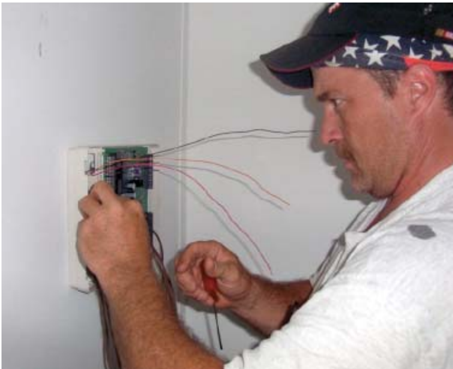
Figure 5. The “user interface” circuit board is the brain of the comfort system; it continually adjusts the air handler, outdoor heat pump, and zone dampers based on sensor input and its programmed instructions. The board shown, a Bryant Evolution control, is capable of managing a wide variety of mechanical systems and can serve as many as eight independent zones.
