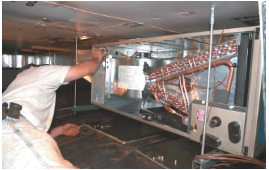
Figure 3. Inside the house, the author installs a variable-speed air handler that is matched to the outdoor condenser. Controlled by advanced electronic circuitry, the air handler's motor can continually adjust to changing loads, ramp up and down gradually as needed, and even sense and adjust to changes in static pressure in the duct system.
