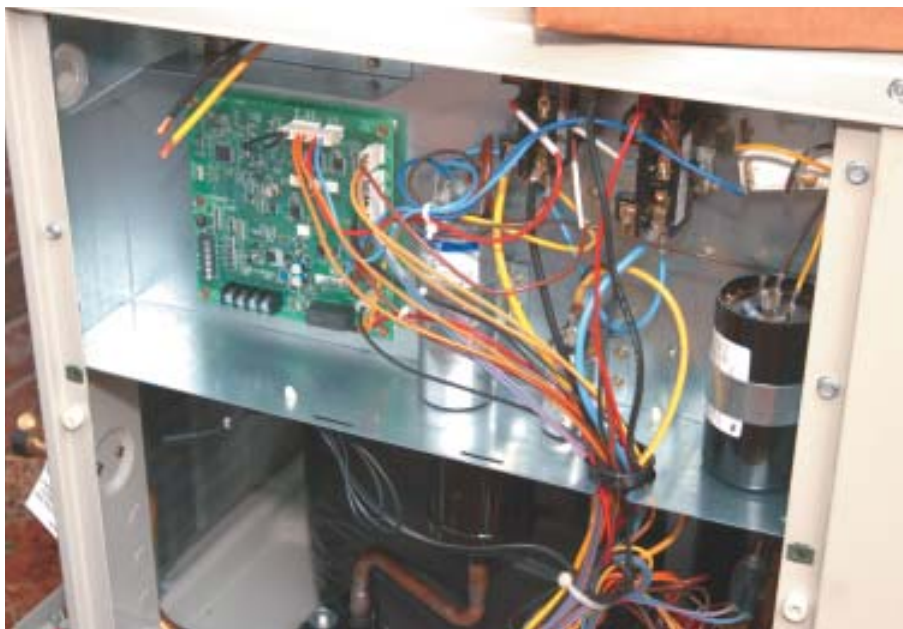
Figure 2. Bryant's top-of-the-line Evolution heat pump has a two-speed compressor controlled by a dedicated circuit board. The compressor experiences fewer on/off cycles than one-speed models, operating at low speed for most of its service hours, and achieves 15-SEER cooling performance with effective dehumidification. Other manufacturers have comparable systems that adjust to low-load or part-load situations.
