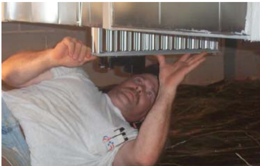
Figure 4. The author likes to zone heat pump or air conditioner setups using zone dampers within the ductwork, controlled by the same master circuit board that manages other aspects of the system. If one zone requires more or less cooling or dehumidification, the master controller can address that zone's needs independently of other zones.
