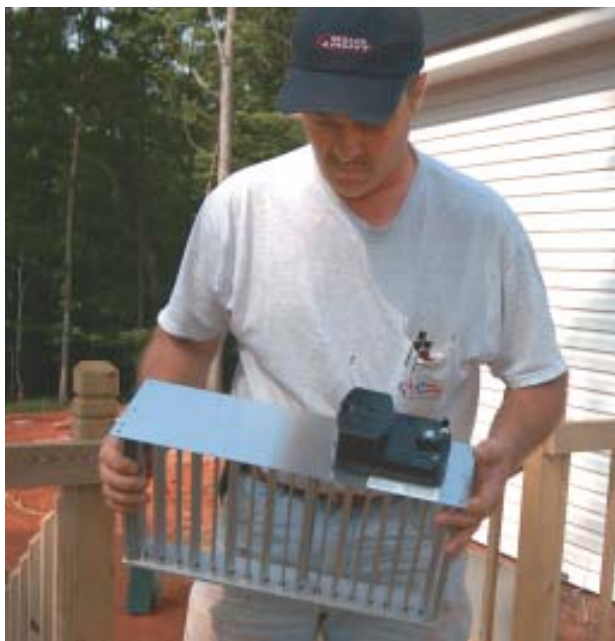
Figure 4. The author likes to zone heat pump or air conditioner setups using zone dampers within the ductwork, controlled by the same master circuit board that manages other aspects of the system. If one zone requires more or less cooling or dehumidification, the master controller can address that zone's needs independently of other zones.
