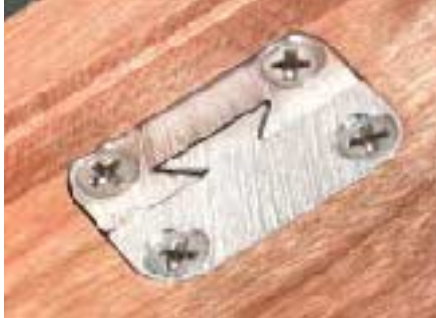
Figure 4. Manufacturers use different techniques to strengthen their frames. For instance, Weather Shield uses interlocking dovetails and side locks to keep double-hung sash in place.
