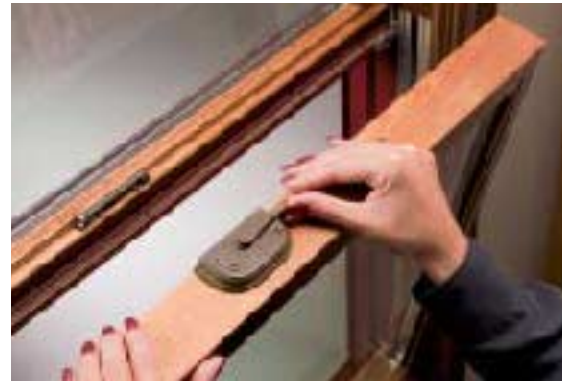
Figure 3. Glass is just half the story. Heavy-duty hardware is supposed to prevent cycles of extreme positive and negative air pressure from pulling a window out of its frame.
