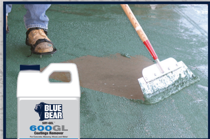
Removal of Floor Paint
