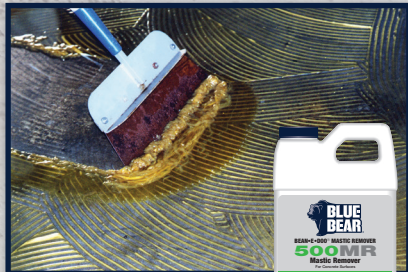
Removal of Vinyl Mastic
